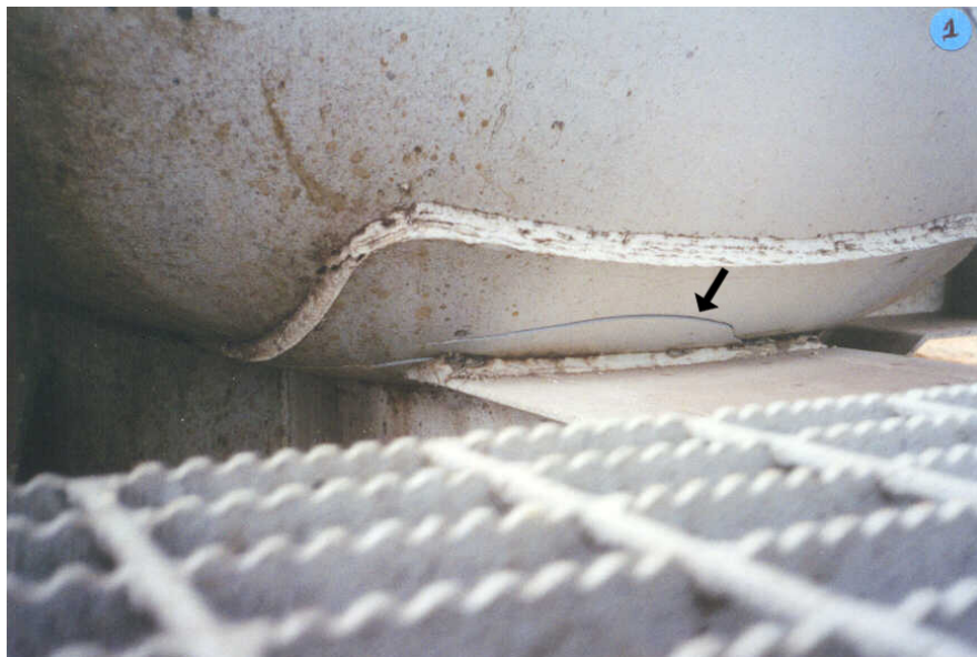
Figure 1. A Sill Pad on a Tank Car–The Arrow Points to a Crack that Was Caused by High Coupler Forces Resulting from an Over-Speed Impact
