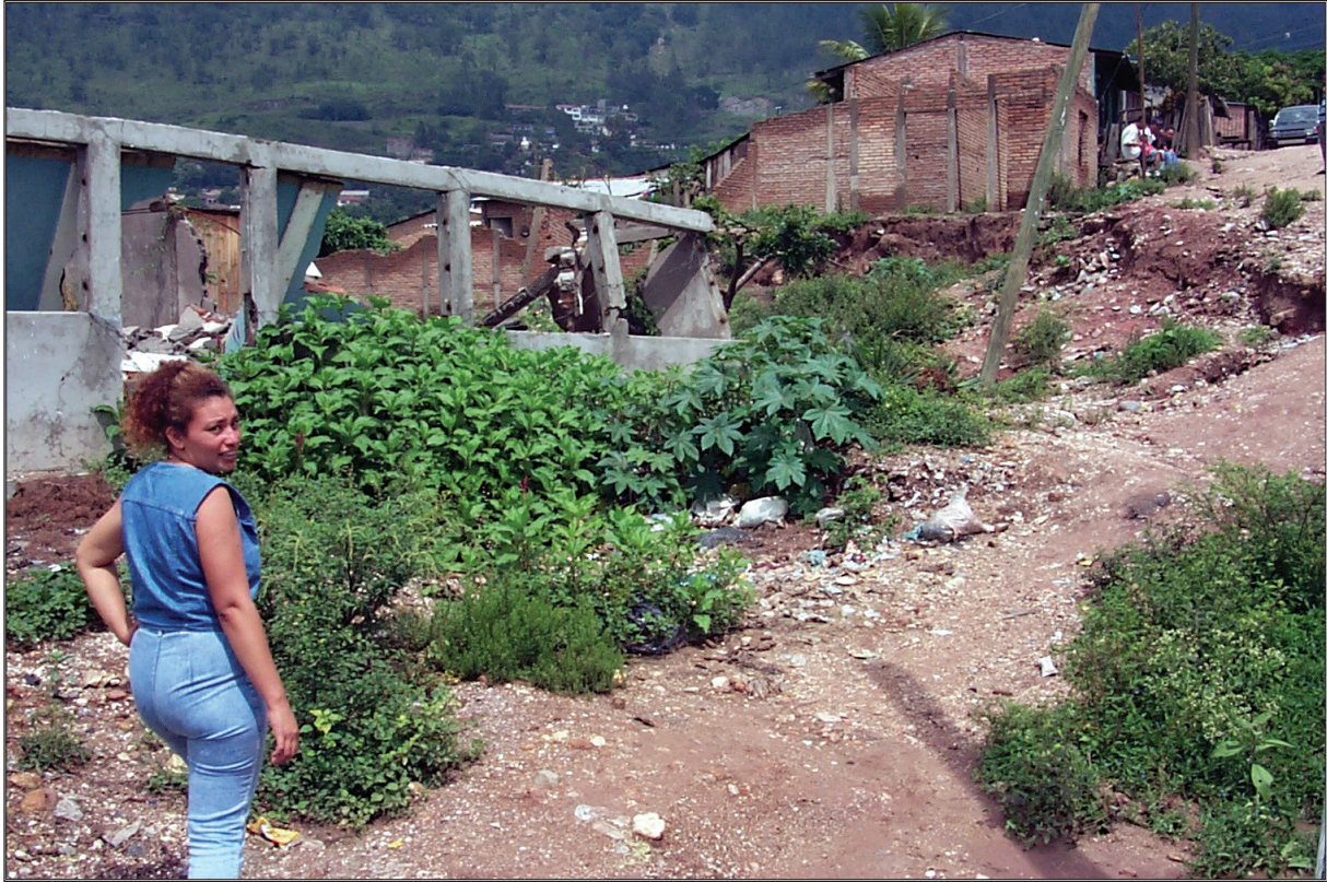
Figure 10. Reactivated slump in Barrio Santa Rosa triggered by intense rainfall in September 1999.
