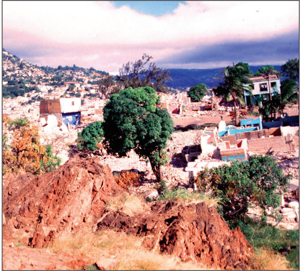
Figure 3. View of the highly deformed toe area of the El Berrinche landslide that destroyed Colonia Soto. The view here is of the remains of Colonia Soto as seen in December 1998. The remains of houses and streets can be seen rotated at high angles from horizontal.
