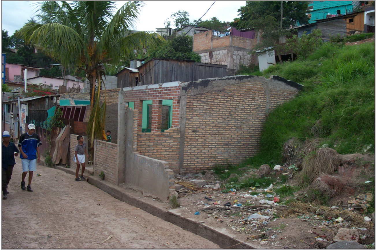
Figure 11. Toe of slump in neighborhood of Campo Cielo in Tegucigalpa. At the right of the photo, the toe of the slide mass is seen impinging against the row of houses.
