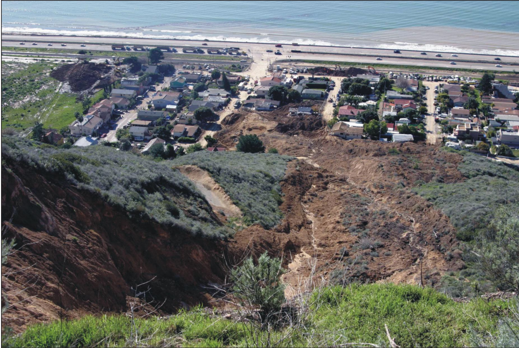
Figure 6. View from the main scarp down the length of the 2005 La Conchita landslide. Water visible in the center of the photograph was issuing from the base of the main scarp when the photograph was taken (January 14, 2005). The 2005 landslide remobilized about 15 percent of the 1995 deposit and followed the left margin (looking downslope) of the 1995 slide. The vegetated ridge in the left part of the photograph is intact material that did not fail in 1995 or 2005; the material in the right part of the photograph is 1995 deposit that is still in place.
