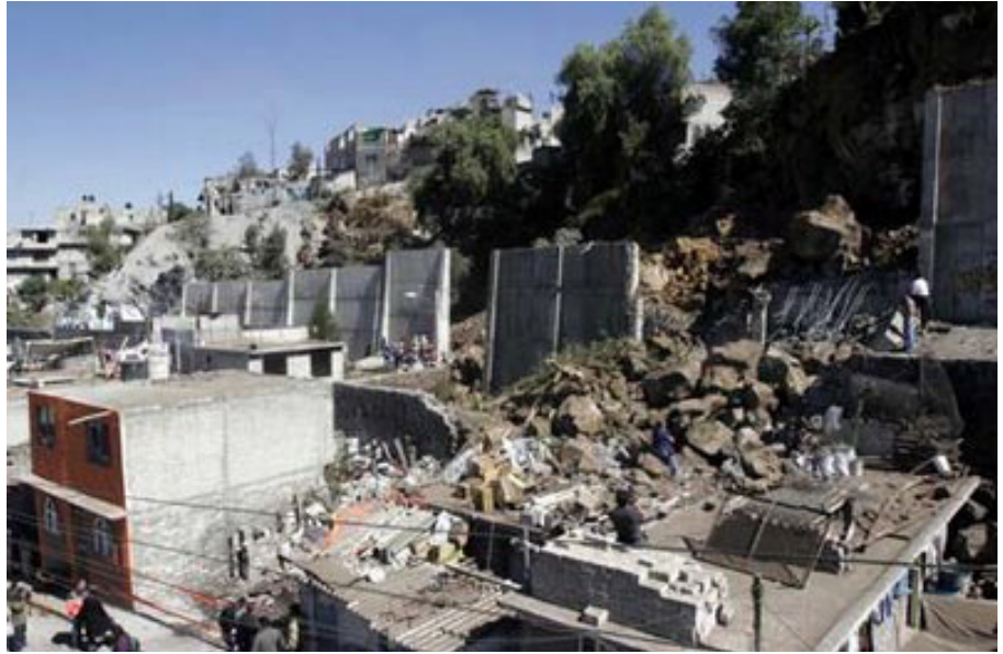
Figure C36. Caution is required in locating and constructing debris-flow retaining walls. This is a photograph of the partial failure of a retaining wall, caused by a landslide in Iztapalapa, a suburb of Mexico City, Mexico. The landslide slid onto a house at the toe of the slope, killing two people, and was triggered by heavy rains in the area. The house was below the 5-meter-high (15 yards) wall, but the wall could not withstand the mass of rocks and soil. (Photograph by Chinagate/Xinhua.)
