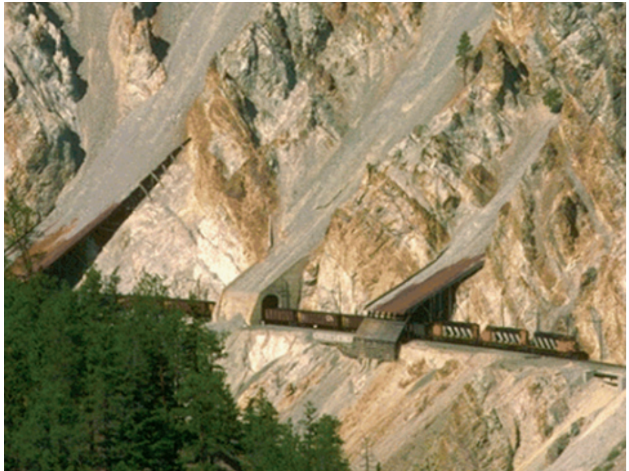
Figure C24. Pitquah rock sheds, British Columbia, Canada. These sheds enclose sections of railroad, protecting it from rockfall and rock avalanches. (Photograph by John Carter, www.trainet.org .)
