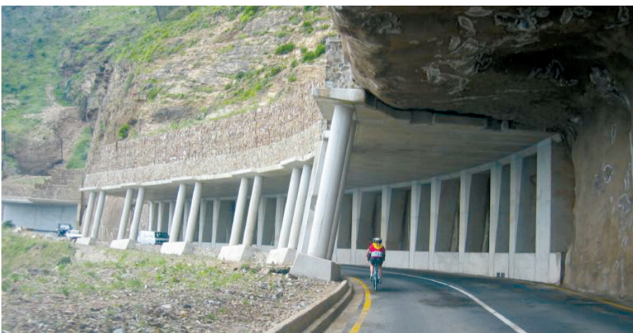
Figure C27. Example of a reinforced rock ledge, Chapmans Peak Drive, Cape Town, South Africa. Photograph attribution: http://commons.wikimedia.org/wiki/Image:Chapmans_peak_dr.jpg .
