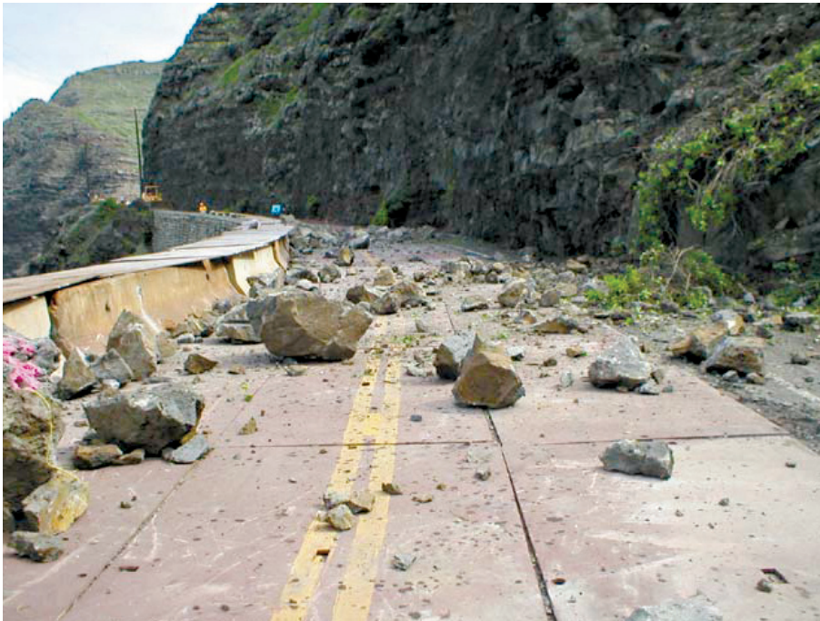
Figure C29. Rocks dislodged by scaling and blasting. (Photograph by Washington Department of Transportation, USA.)
