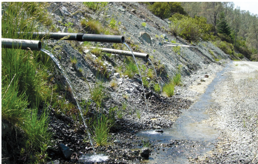
Figure C10. Schematic of drainpipes. (Schematic from Reference 11.) Photograph of drainpipes in a landslide in California, USA, by Andrew Alden.
