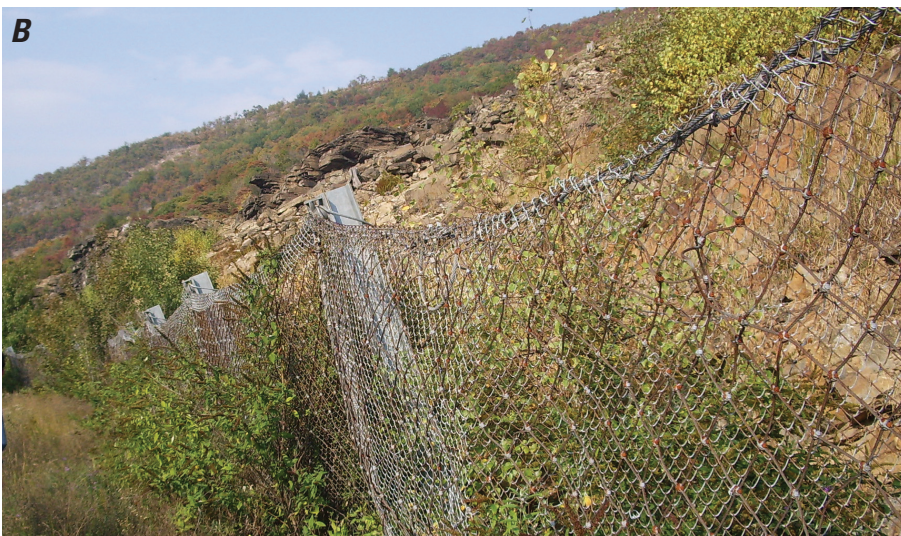
Figure C22. Protective rock barrier fencing along (A) a dirt trail in Pennsylvania, USA, and (B) a roadway in coastal California, USA. (Trail photograph, Lynn Highland, U.S. Geological Survey; roadway photograph from Federal Highway Administration, USA.)
