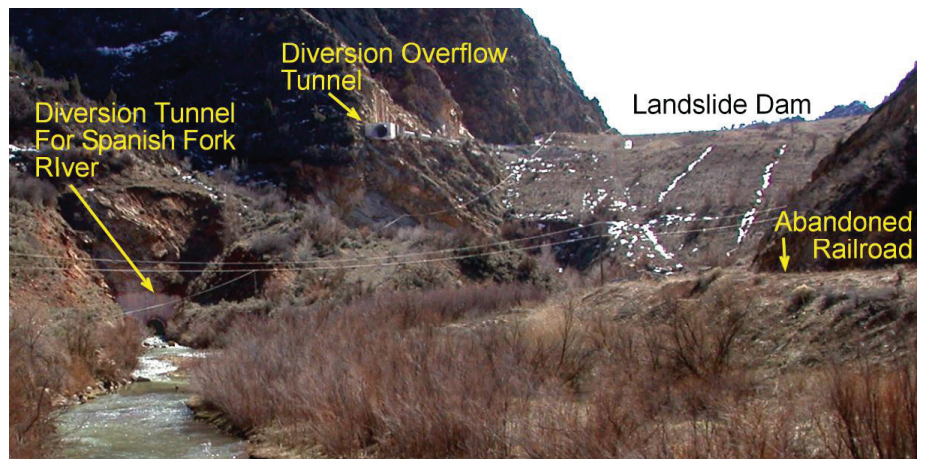
Figure C54. Closeup view of mitigation measures taken to reduce the impact of the Thistle landslide dam, showing the tunnel for the river, and the diversion overflow tunnel. (Photograph courtesy of the Utah Geological Survey).
