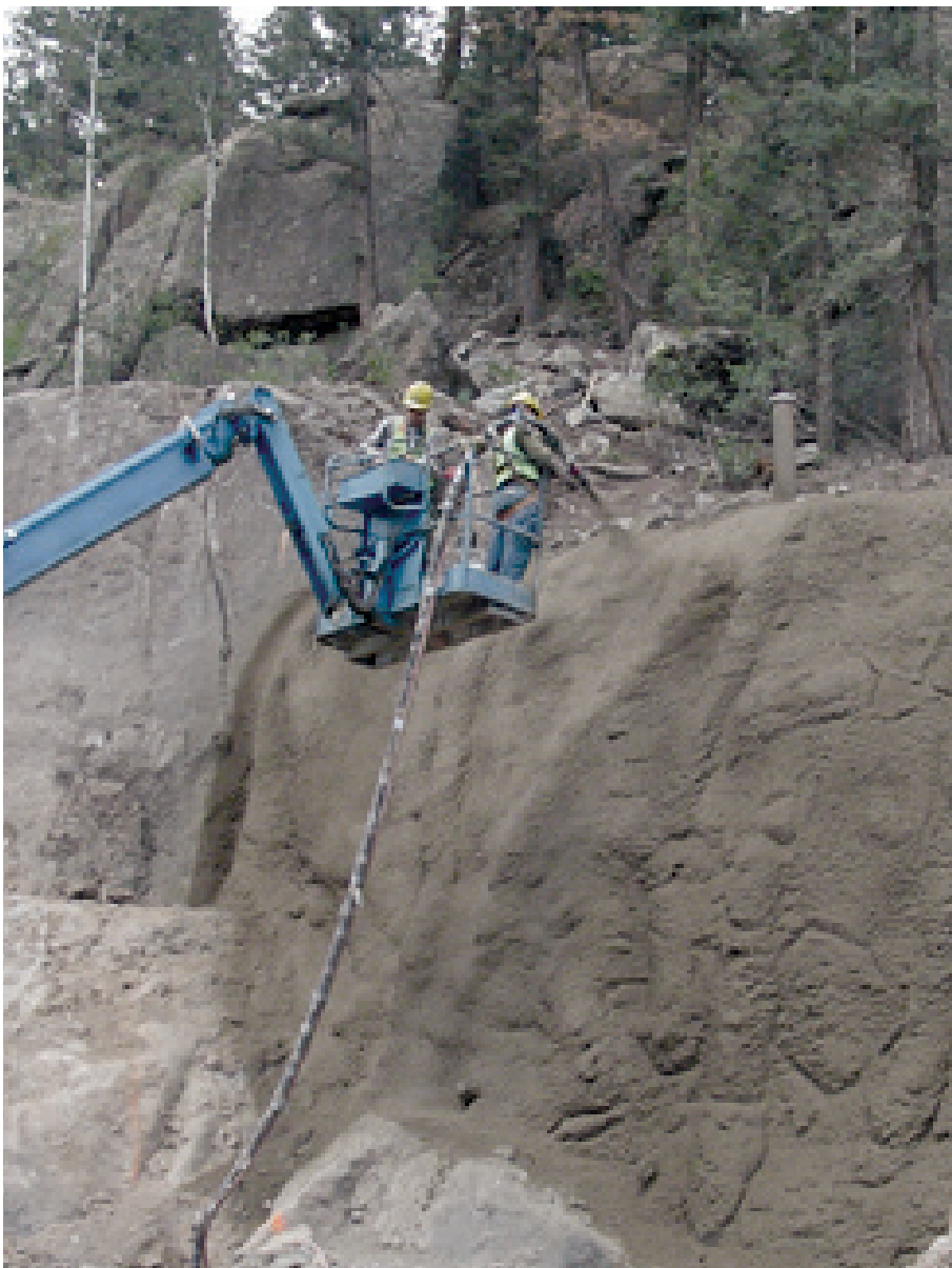
Figure C31. Shotcrete operation to stabilize rockfall area of Wolf Creek Pass in the Rocky Mountains of Colorado, USA. (Photograph by Colorado Department of Transportation.)
