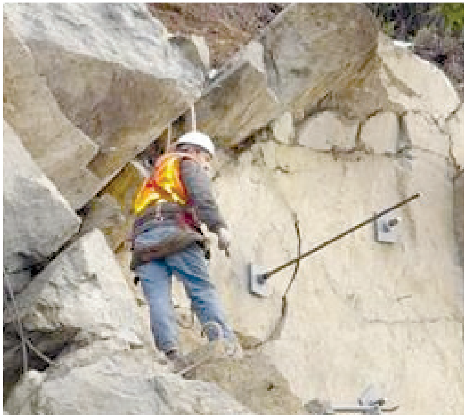
Figure C33. A rock bolting operation; notice broken-up (crumbling) nature of the rock. (Photograph by Washington Department of Transportation, USA.)
