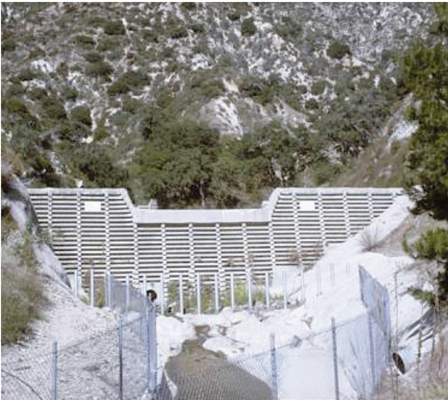
Figure C8. Upstream view of concrete crib-type check dam with low-flow center section in southern California, USA. (Photograph by Los Angeles County Flood Control District.)
