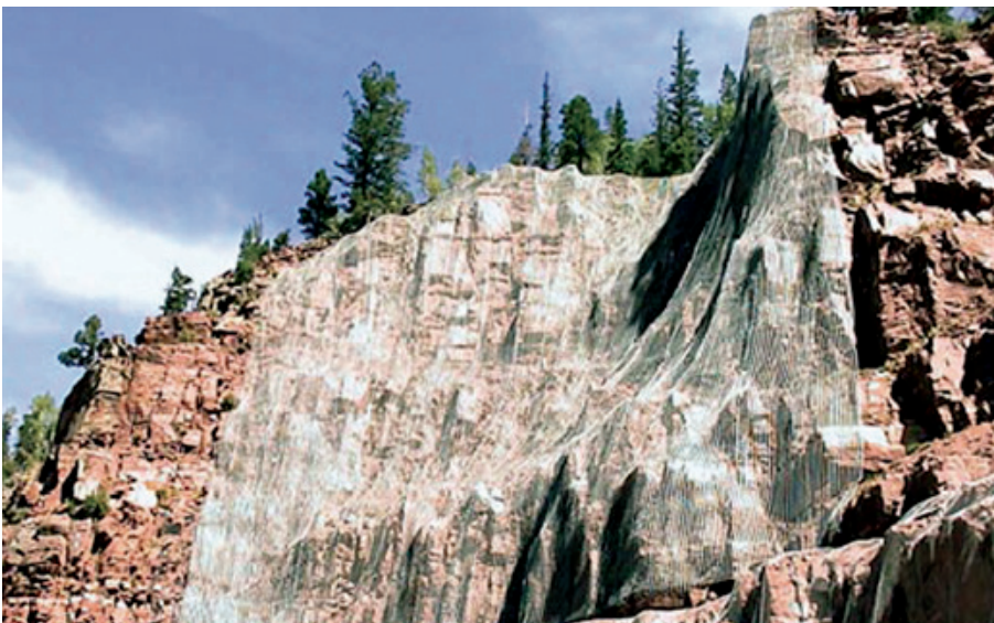
Figure C23. Example of a "rock curtain" that controls rockfalls in problem areas. (Photograph by Doug Hansen, High Angle Technologies, Inc.)
