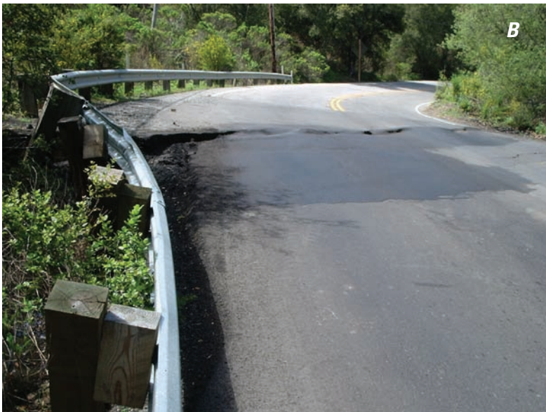
Figure 5. Sites of slope movement on the Weeks Creek landslide (fig. 1) during California water year (July 1–June 30) 2005–6. A, Lateral and vertical displacements at northern margin of landslide near intersection with California Highway 84 on April 26, 2006. B, Lateral displacement of roadway at southern margin of landslide on April 28, 2006. Photograph by Katerina Rousseva, graduate student at San Jose State University. C, Slight new ground cracks within east side of prehistoric section of landslide on May 31, 2006.
