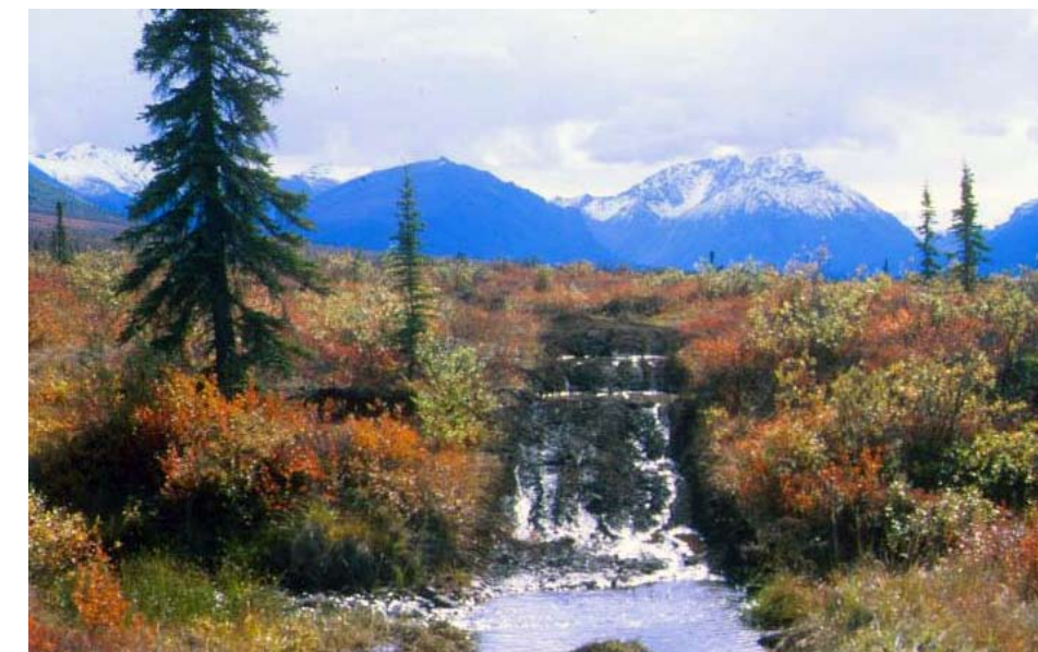
Damage on the Copper Lake Trail caused by ORV use. Fragile tundra and permafrost are not the ideal substrate to build a trail on. Mudholes cause an impassable trail during wet times of year. Users eventually just go around the mudholes creating a wider, more braided trail that impacts a larger area of the Park.
