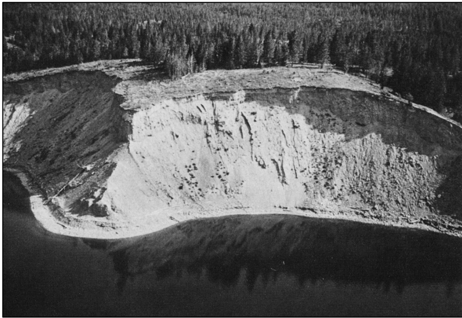
Figure 31. Bluff consisting of mostly non-cohesive sand and gravel undergoing failure by individual grain falls and shallow, localized slips. Material accumulates at the base as talus deposit, which protects the slope from further undercutting and failure until removed by waves and currents.
