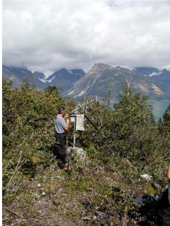
Figure 3. GOES test site in Queen Inlet. GOES satellite transmission system transmits hourly data on precipitation and air temperature, while also storing these data as a backup on Campbell data logger located within the grey box.
