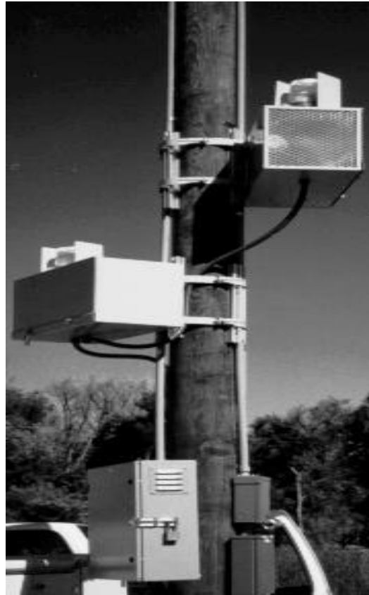
Figure 2. Wayside Horn on Utility Pole
