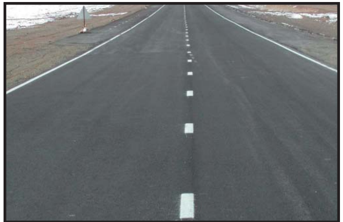
Photograph of the Kabul-Kandahar Highway, with striping and signage, near Km 48.
