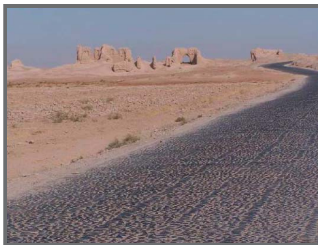
Photograph of a cobblestone farm-to-market road built under the cash-for-work program.
