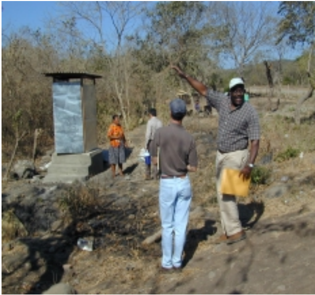
OIG team inspects a USAID-sponsored latrine project at Hato Nuevo community.
