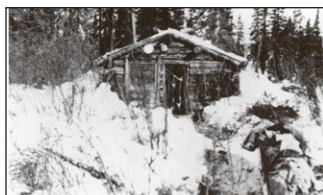
4-Mile Trapper Cabin
