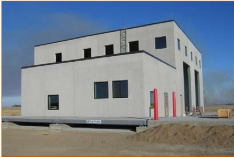
Figure 23: Transfer station near completion.
