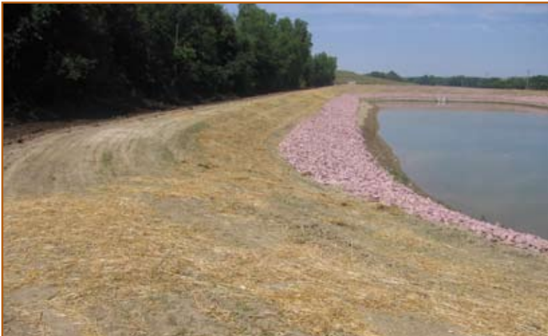
Figure 17: Completed settlement pond cell with riprap.
