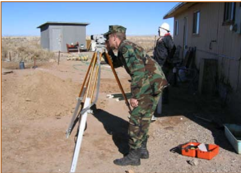
Figure 38: Engineer Kurt Kesteloot surveying to ensure the drainfield line is level.
