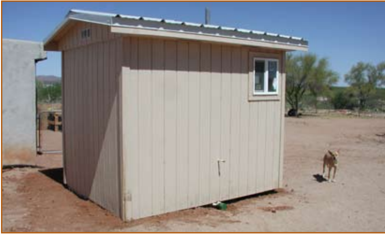
Figure 31: Back of modular bathroom.
