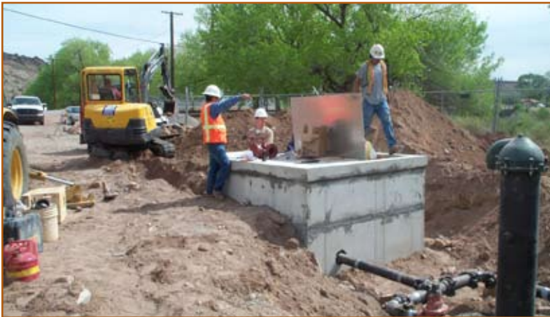
Figure 33: Engineer Quentin Allen inspecting the construction of booster station, NM.
