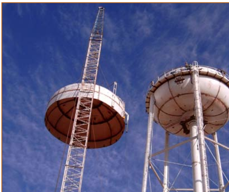
Figure 27: Construction of the elevated water storage tank.
