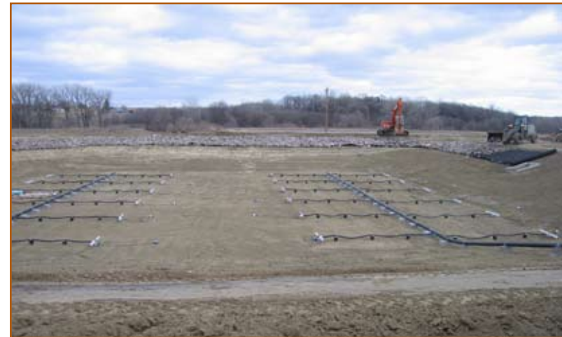
Figure 18: Aeration diffuser piping placed on bottom of aeration cell.
