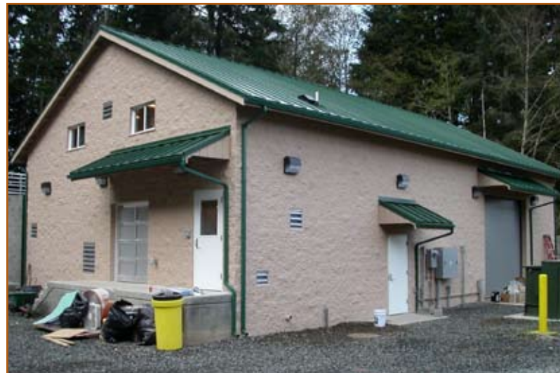
Figure 16: New Makah WTP near completion.
