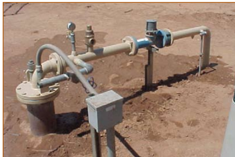
Figure 28: Upgraded well pumps and piping.
