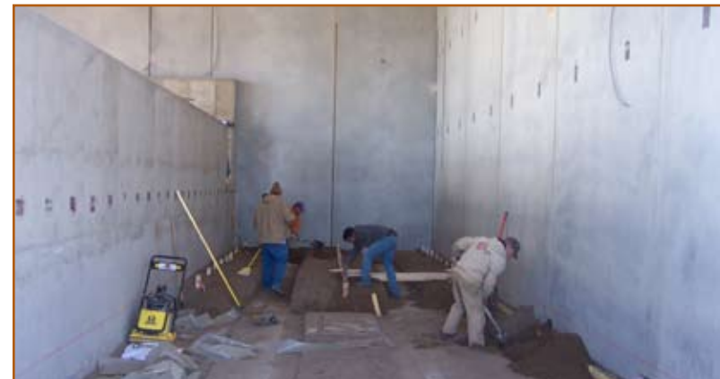
Figure 22: Workers prepare for concrete pour in transfer station load-out area.
