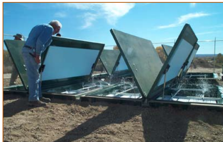
Figure 8: Startup of an Advantex water reclamation facility serving 20 homes, NM.
