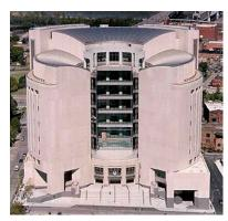
The roof replacement project at the Whittaker Courthouse started in late spring 2008 and will be complete in April 2009. The project consisted of the complete removal of the original roof system down to the concrete deck on all the roof areas.
