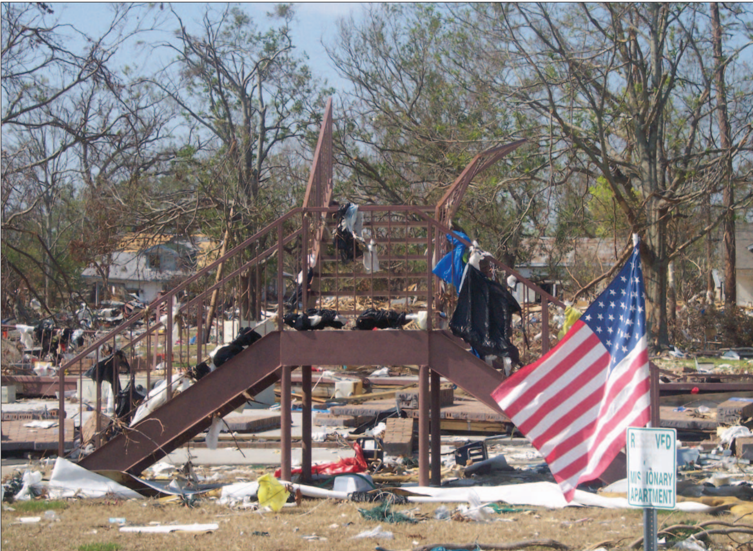
Ruins of apartment building, Long Beach, MS Denton Herring photo
