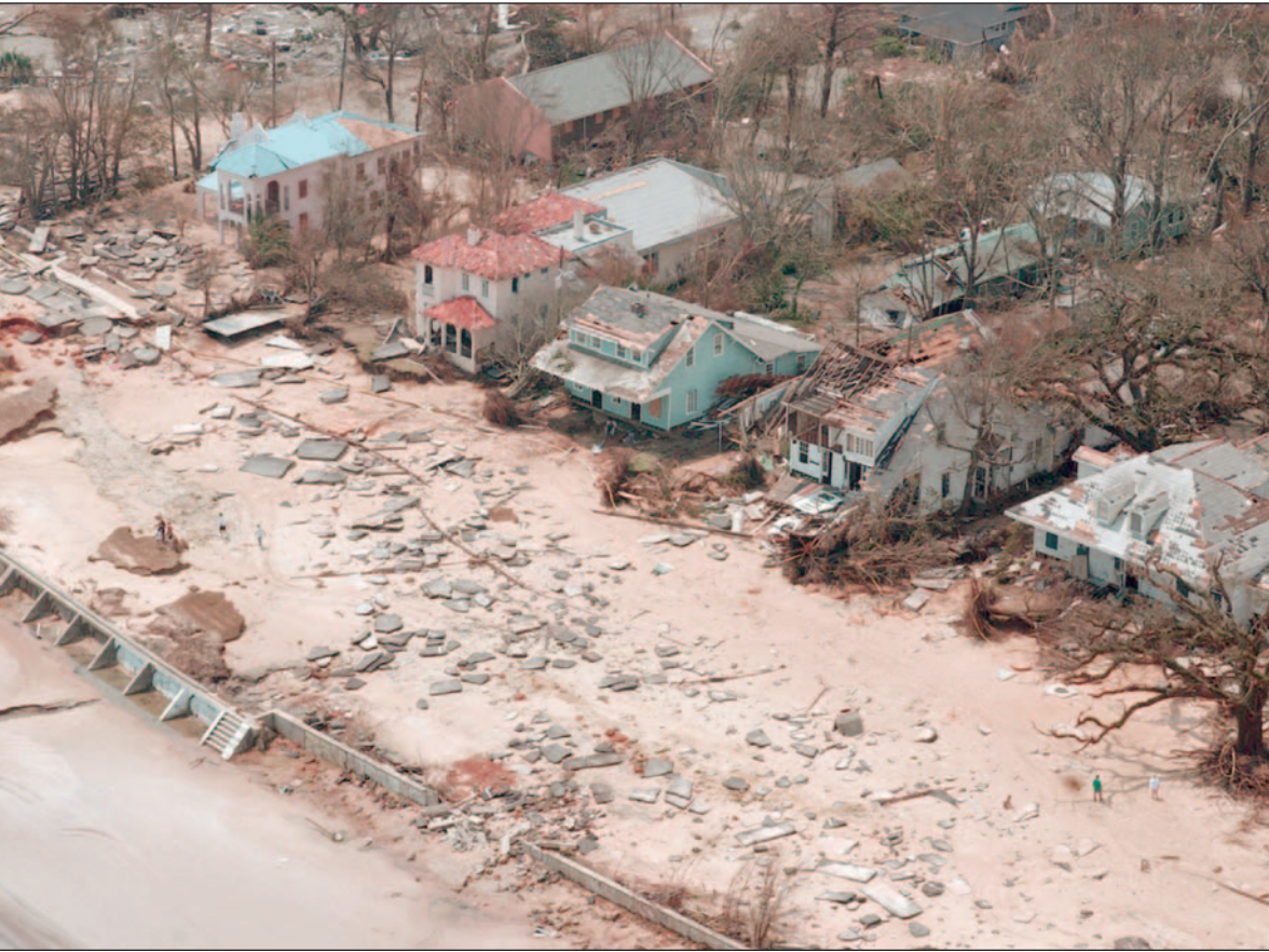
Ruined homes, Bay St. Louis, MS Sun Herald news photo, Biloxi/Gulfport, MS
