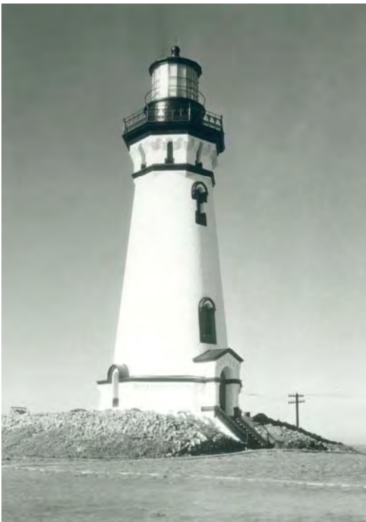
The lighthouse prior to removal of the top portion.
