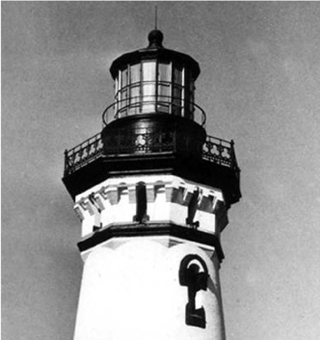
Close up view of the top of the light house circa 1932.
