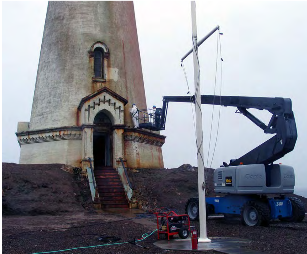
Conducting structural testing on the light house in 2006.
