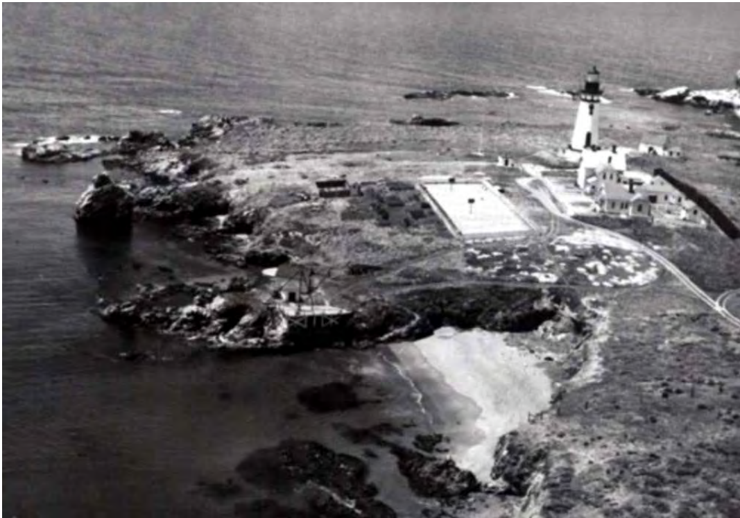
The rain catchment area (rectangular slab) is clearly seen in this old photo, along with the wharf.
