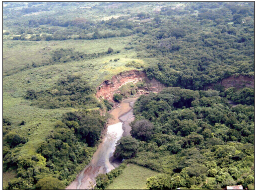
Figure 18. Bank failure on the Río Gualcho about 4 km upstream of Embalse 15 de Septiembre. This and similar failures along the Río Gualcho may have resulted from accelerated bank erosion cause by the high stream flows that occurred during Hurricane Mitch.
