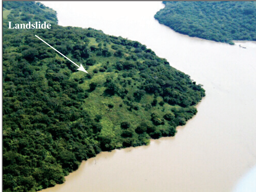
Figure 16. Large dormant pre-hurricane landslide on the shore of Embalse 15 de Septiembre. If reactivated, a large landslide such as this one might partially block the reservoir, however, it is far enough upstream from the dam that it probably would not interfere with operation of the dam or the hydroelectric facilities.
