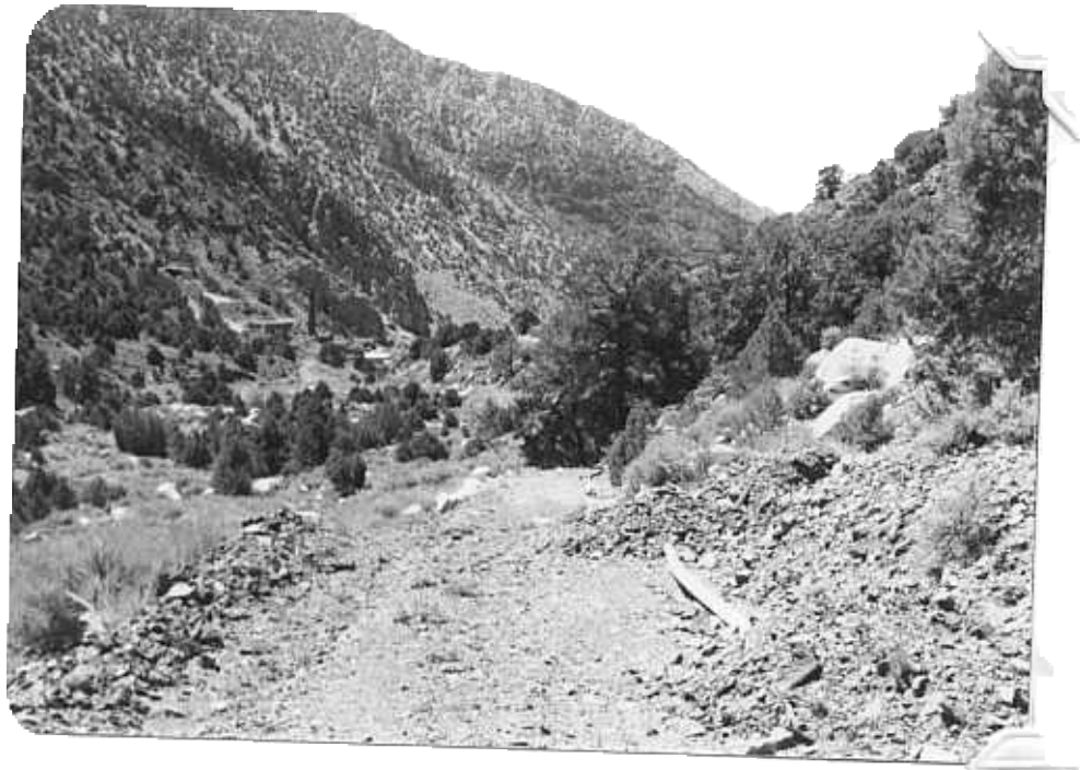
Figure 11. Partially buried water line leading toward Mineop Corp. facilities near Panamint City.
