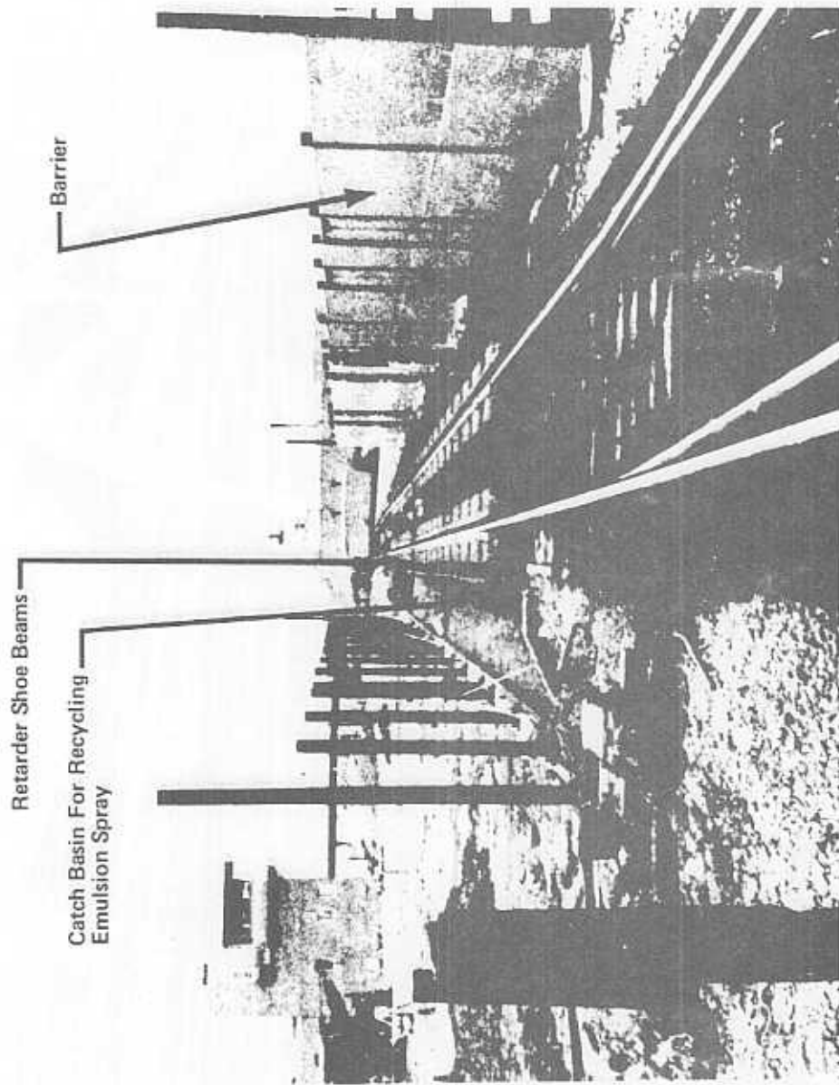
FIGURE 2.2 VIEW, NORTHERLY FROM EXIT END OF GROUP RETARDER NO. 3, WITH WESTERLY BARRIER WALL REMOVED
