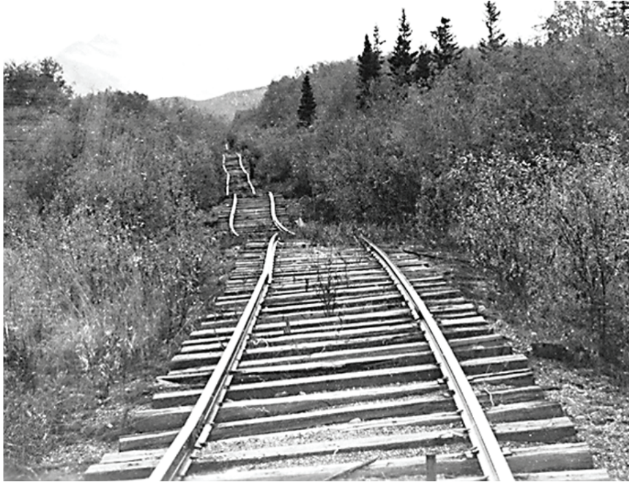
Figure 2.11. Abandoned railroad tracks warped by thermokarst near Valdez, Alaska. During construction of the roadbed the thermal equilibrium of the permafrost was disrupted causing differential thawing.
