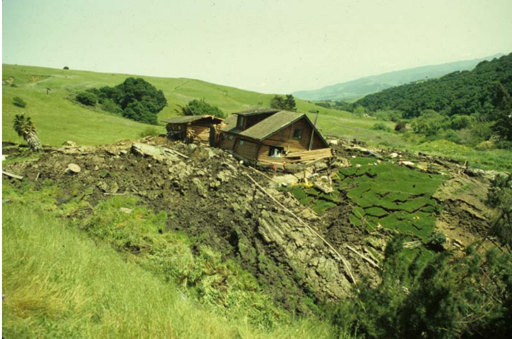
Figure 1A. Deep-seated rotational slump in San Benito County, California, that has broken a natural gas pipeline. Landslide was triggered by rainfall from El Niño conditions April 22, 1998 (Photo by Robert Schuster, USGS).
