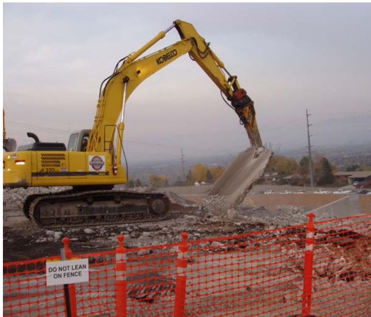
Figure 17. Approach panel removal.
