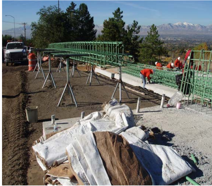
Figure 15. Sleeper slab reinforcement assembly.
