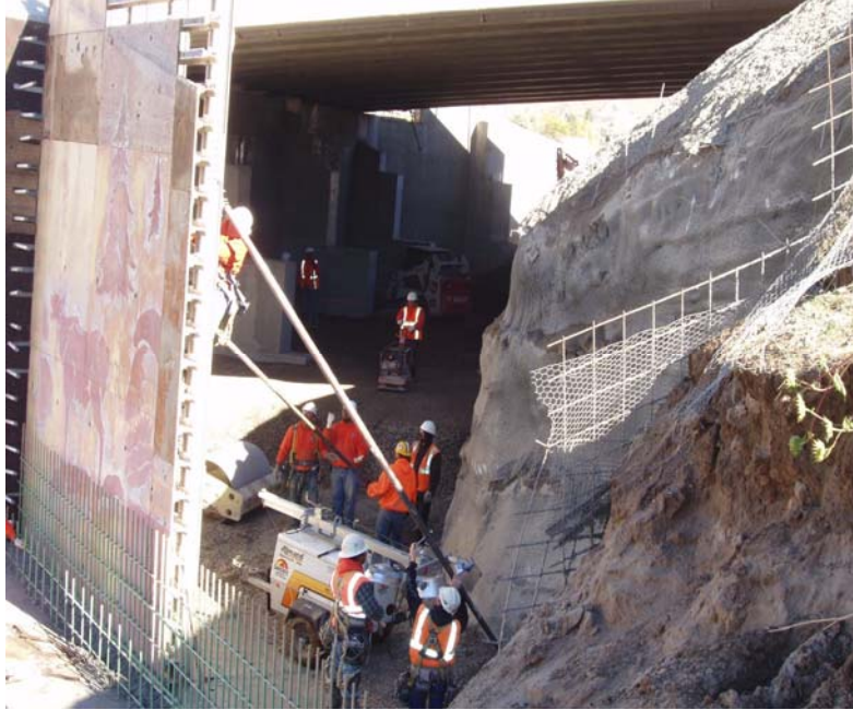
Figure 13. Seating the backfill material.
