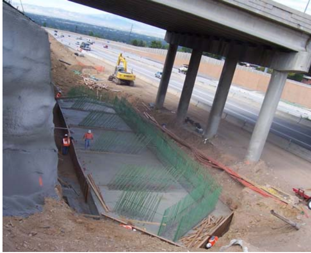
Figure 7. View of the east spread footing.
