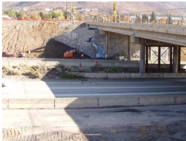
Figure 9. View of CIP wingwall.
