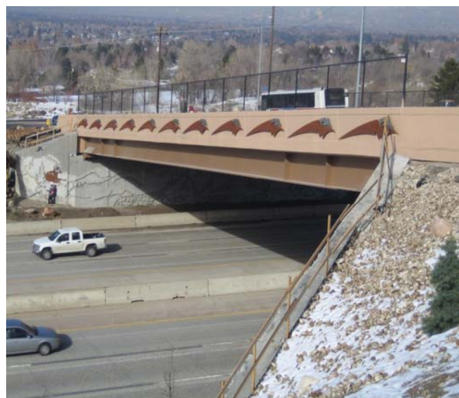
Figure 27. Another view of the new 4500 South Bridge.
