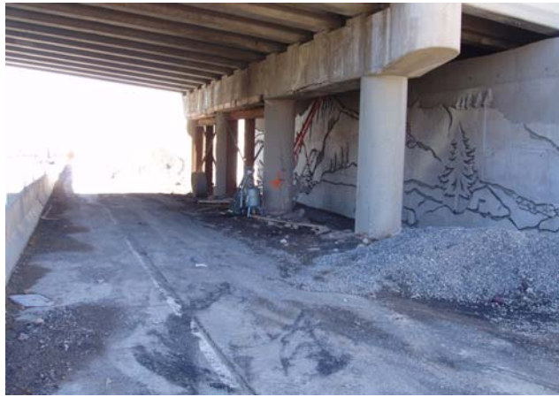
Figure 8. View of the CIP abutment.
