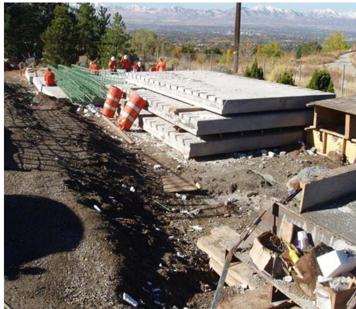
Figure 14. Precast approach slabs.
