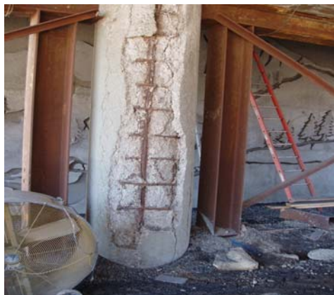
Figure 2. Delaminated column.
