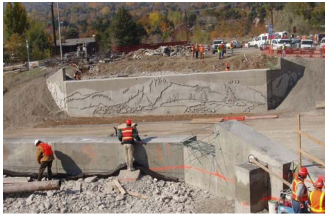
Figure 21. View of abutments and wingwalls with no superstructure.
