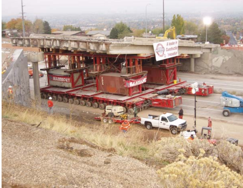
Figure 18. Lifting and removing the first span.
