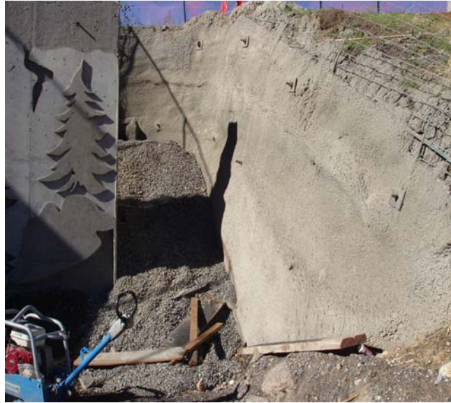
Figure 10. Soil nailing of the approach embankment.
