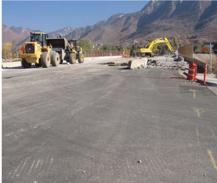
Figure 16. Demolition of railing and median.
