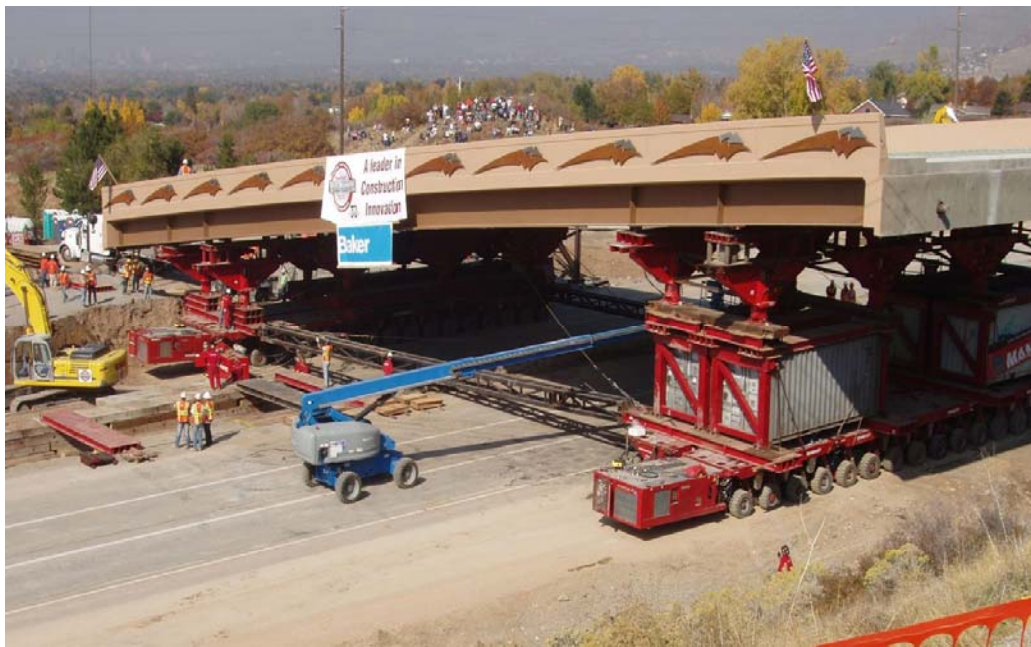
Figure 23. Another view of moving the superstructure.
