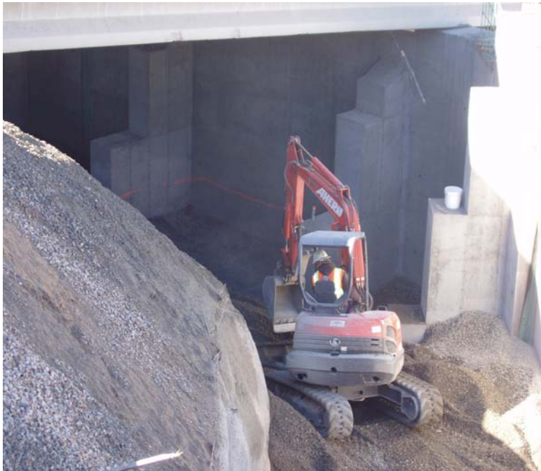
Figure 12. Placement of backfill material.
