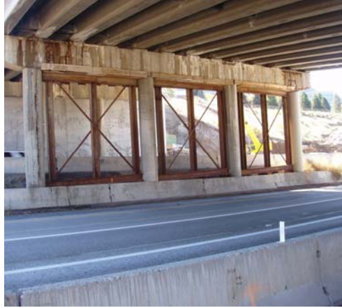
Figure 3. Shoring the bent caps.
