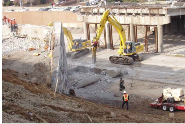
Figure 20. Demolition of the columns and bent caps.
