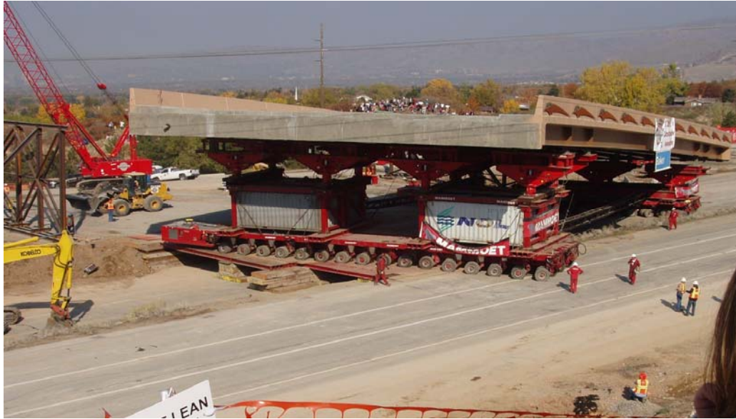
Figure 22. Moving the new superstructure.
