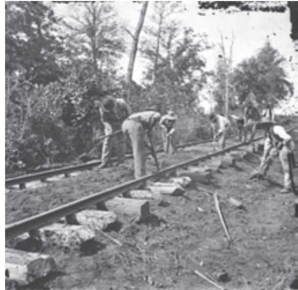
FIGURE 4. Workmen repair the Nashville & Chattanooga Railroad near Murfreesboro after the battle, 1863.
