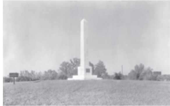
FIGURE 22. View of the Artillery Monument, September 1935.
