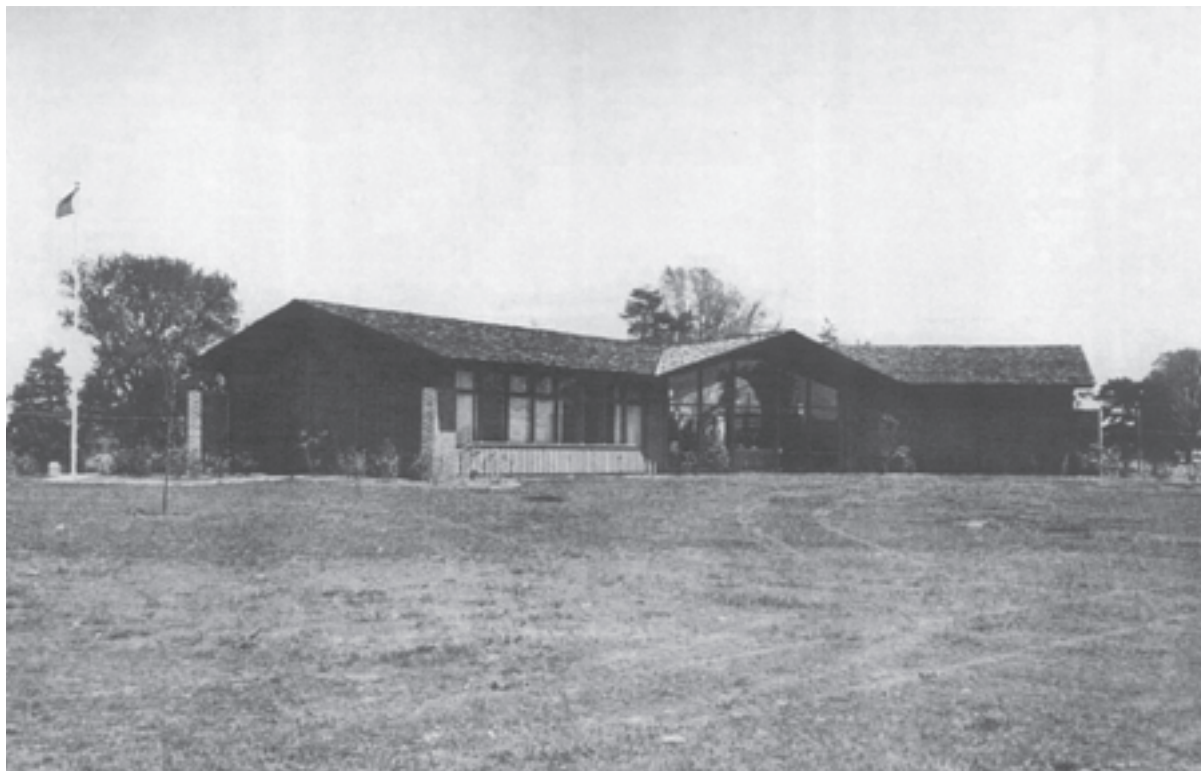
FIGURE 33. View of the newly completed Visitor Center, June 1, 1966.
