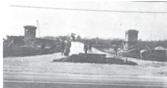
FIGURE 17. The main entrance to the park under construction in 1931.
