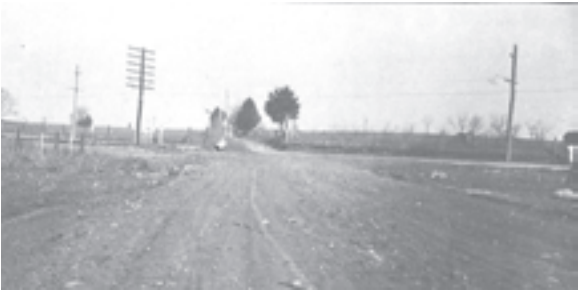
FIGURE 16. Van Cleve Lane in February 1931, after regrading and surfacing by the War Department. This view is looking south across the Nashville Pike intersection.
