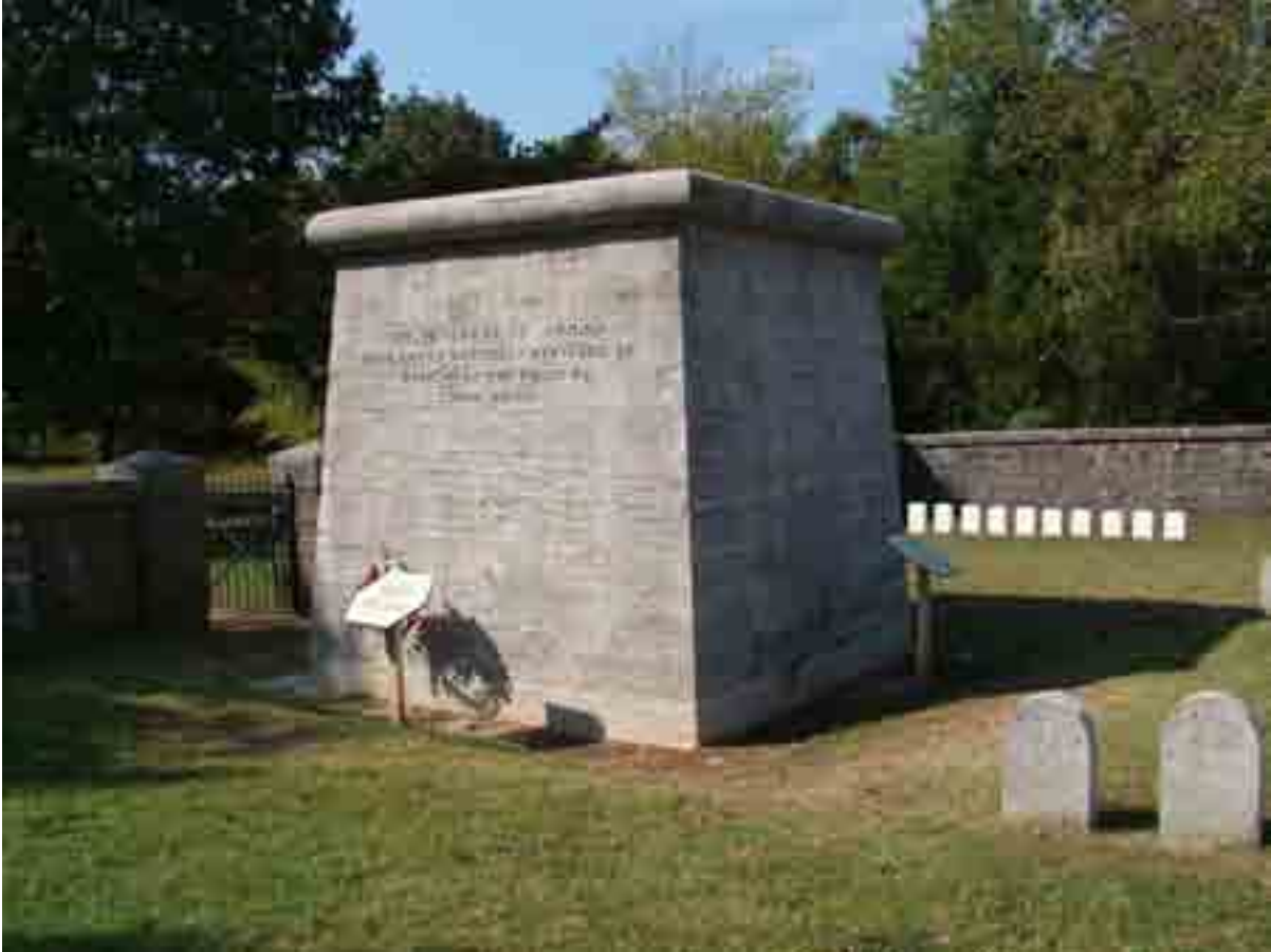
FIGURE 127. Hazen Brigade monument, limestone wall, and metal gate at entrance.
