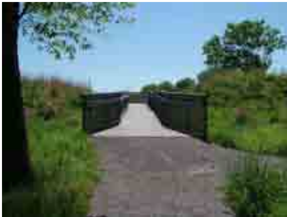
FIGURE 173. Recycled wood and plastic boardwalk leading into the redoubt.
