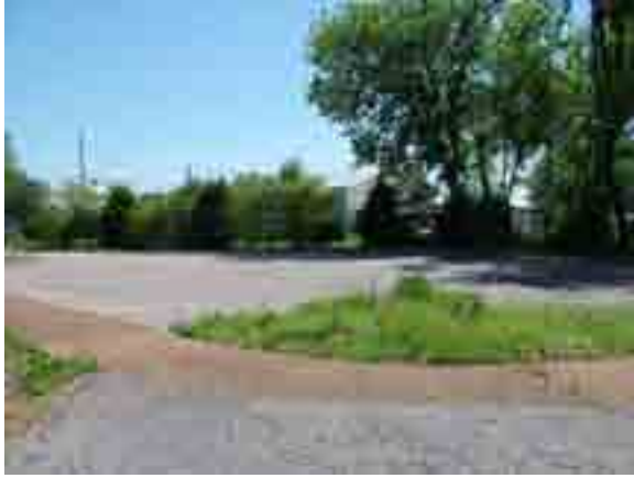
FIGURE 172. Asphalt parking lot.
