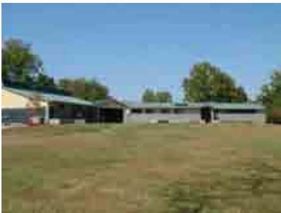
FIGURE 50. View of the visitor center from the southeast.
