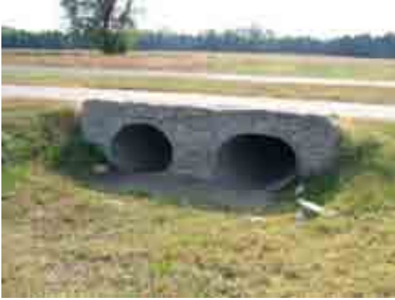
FIGURE 53. Large corrugated pipe culverts with a stone headwall.
