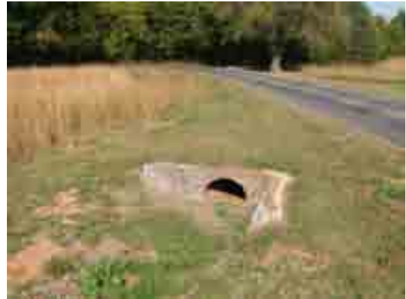
FIGURE 57. Pipe culvert and L-shaped concrete headwall near Tour Road Stop Two.
