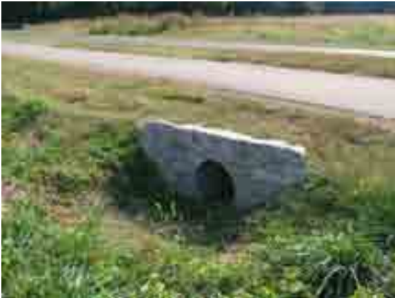
FIGURE 54. Small corrugated pipe culvert with a stone headwall.
