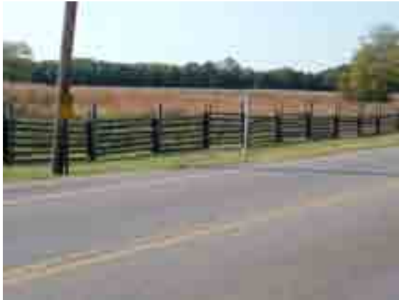
FIGURE 71. Two-post and rail wood fence found between Van Cleve Lane and the visitor center.
