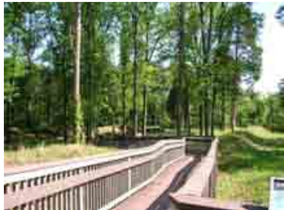
FIGURE 162. Recycled wood and plastic boardwalk at Lunette Palmer.
