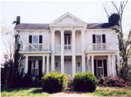
Used as a hospital during the battle of Stones River, the Jenkins House was recently torn down
