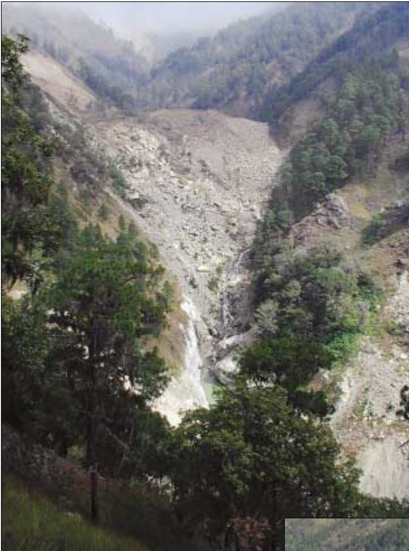
Figure 15. Landslide dam on the Río La Lima, looking upstream (north) from a point 4 km north (upstream) of Jones (see fig. 14); photograph taken 25 January 2000. The landslide originated on the steep slope in the upper left corner of the photograph. The point of discharge of the river from the debris that forms the dam is at the point where the water is first visible at the middle right part of the photograph.
