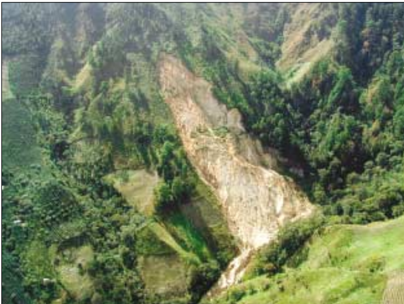
Figure 21. Large landslide on the La Unión quadrangle at UTM coordinates of 245000 E, 1647700 N.
