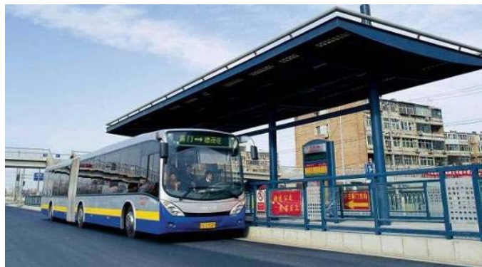
Beijing BRT Line 1 Articulated Vehicle and Station Infrastructure (courtesy of CSTC)
