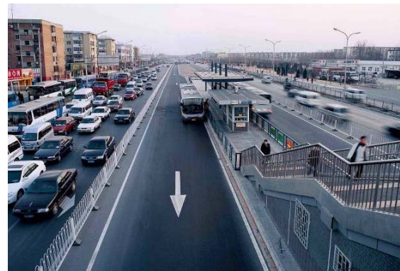
Beijing BRT Line 1 Running Way and Station (courtesy of CSTC)
