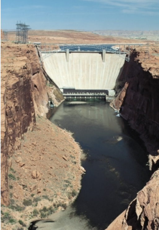
Fig. 10. Glen Canyon Dam, near the Arizona–Utah border.
