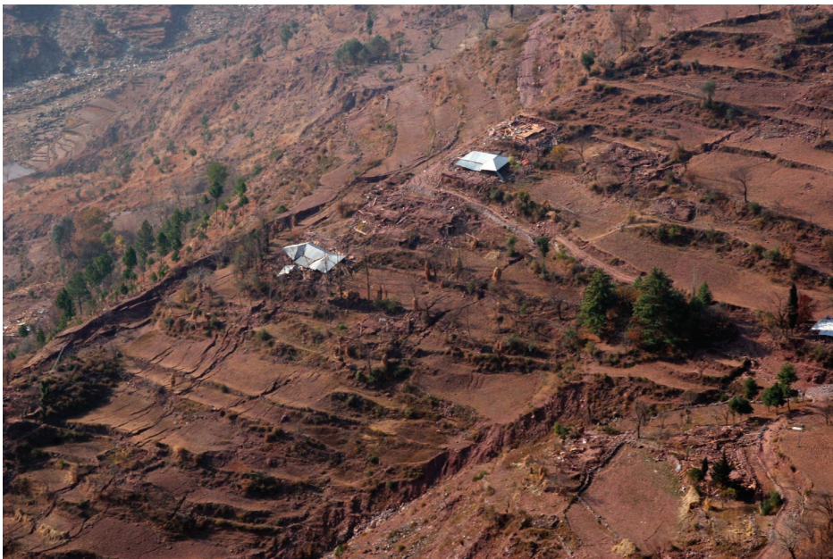
Figure 5. Oblique aerial view of slopes above the reservoir in the Karli stream drainage with numerous fractures (lower left in photograph) extending through the terrain parallel to the slope direction and to the strike of bedding.
