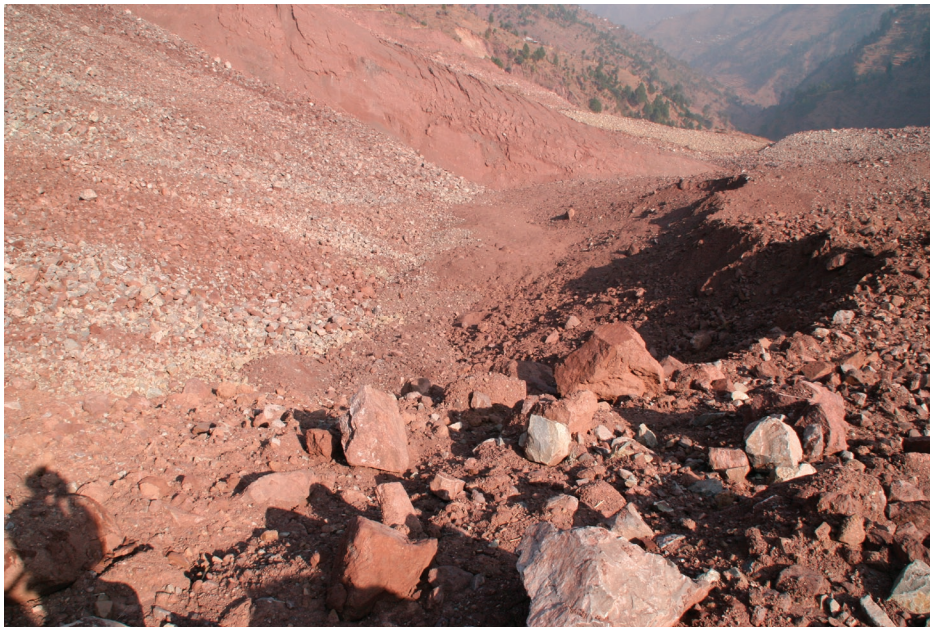
Figure 8. View northeast downvalley from crest of the Karli stream landslide dam where Pakistan military engineers plan to construct a spillway in the debris. Note the depression in the foreground where some of the excavated debris may be deposited.
