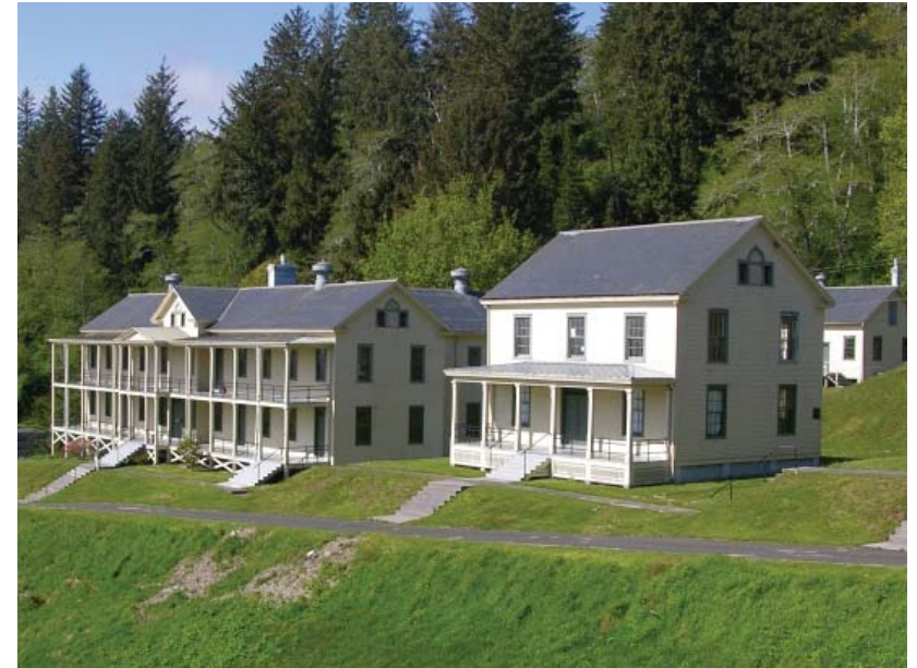
FORT COLUMBIA STATE PARK BARRACKS
