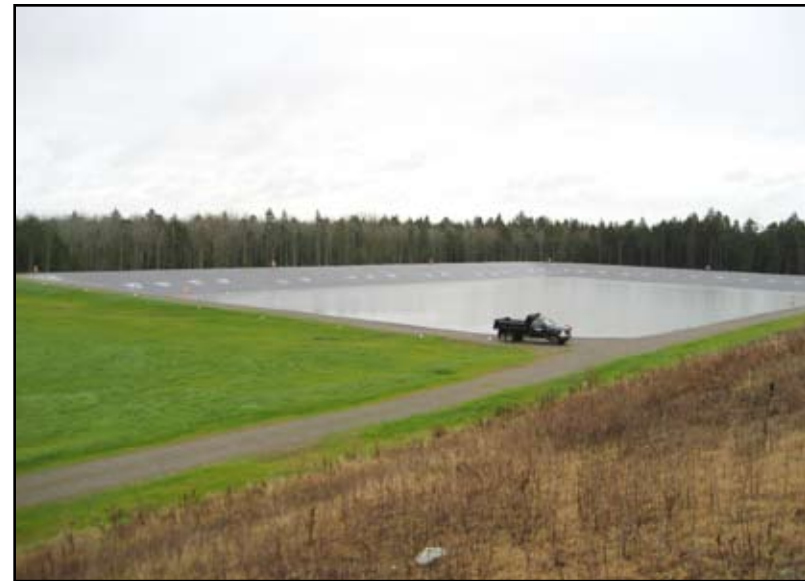
Figure 30: Completed 13 million gallon sewage lagoon for Passamaquoddy Tribe.
