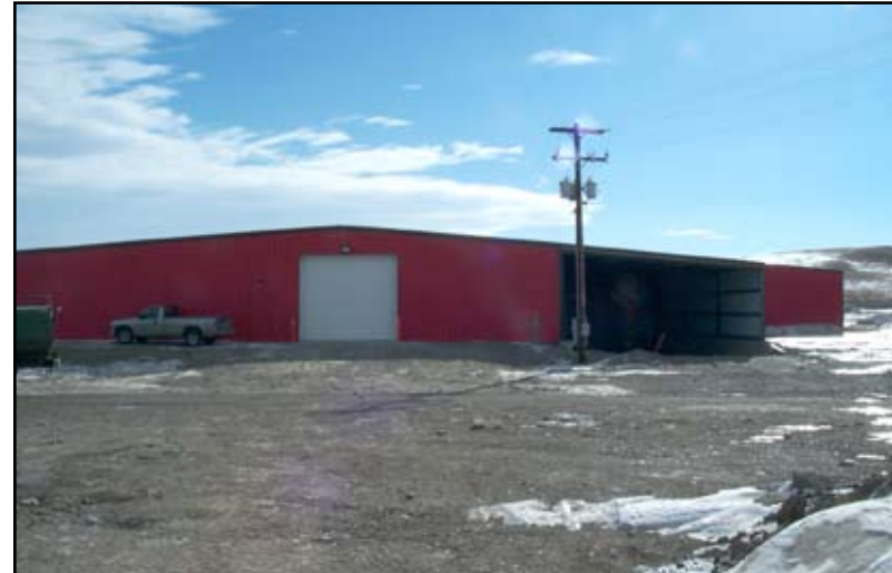
Figure 10: Lumber mill building was remodeled to become the solid waste transfer site.
