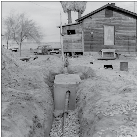
Figure 1: Construction of a septic system, 1960's.
