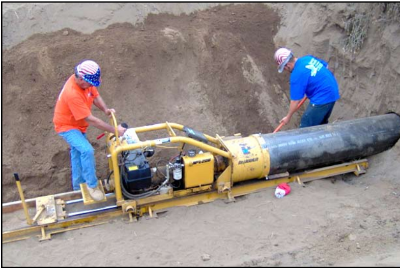
Figure 20: Contractors bore beneath a state highway to install 10" waterline.
