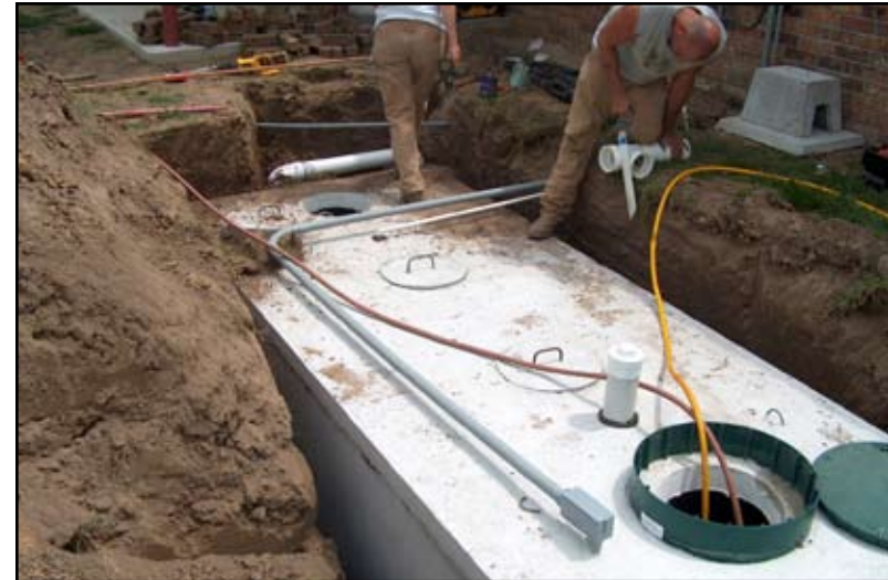
Figure 15: Contractor installing sprinkler system for aerobic wastewater system.
