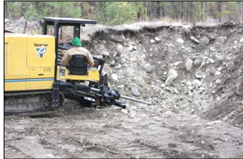
Figure 35: Boring under the San Poil River using horizontal directional drilling equipment for Keller community waster system improvements, Colville Reservation.
