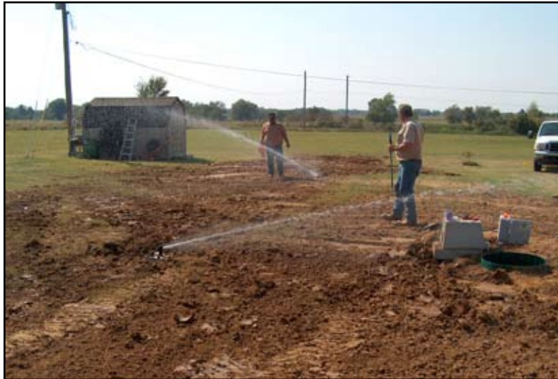
Figure 14: Contractor adjusting sprinkler heads for an individual aerobic wastewater treatment disposal system.
