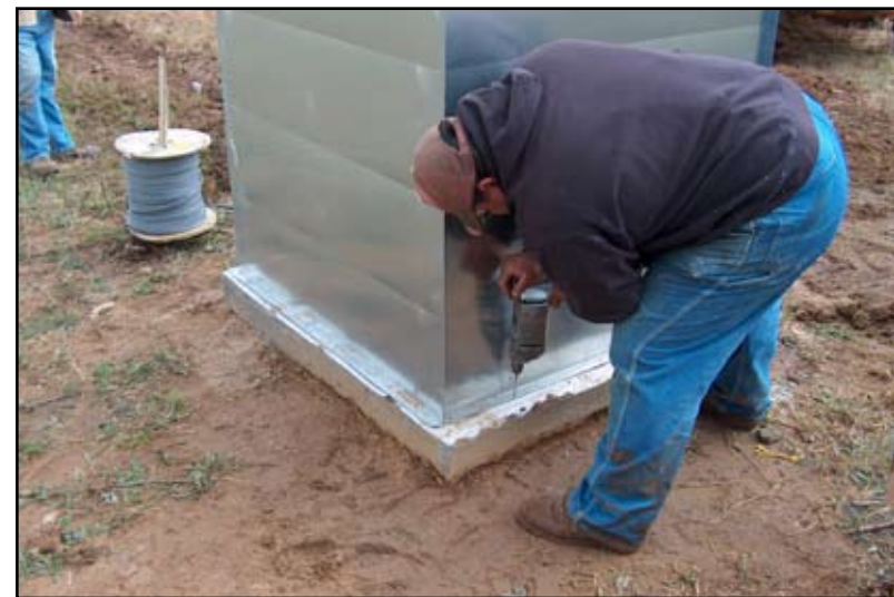
Figure 16: Okmulgee crew member installing a new well house.
