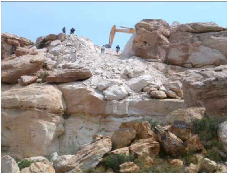
Figure 31: Construction of sewer outfall line for Village of Shungopavi, Hopi Reservation.
