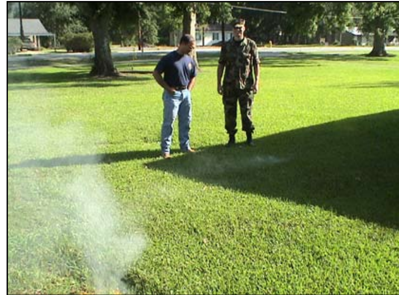
Figure 25: IHS engineer inspecting the smoke testing which identifies infiltration into the wastewater collection system.
