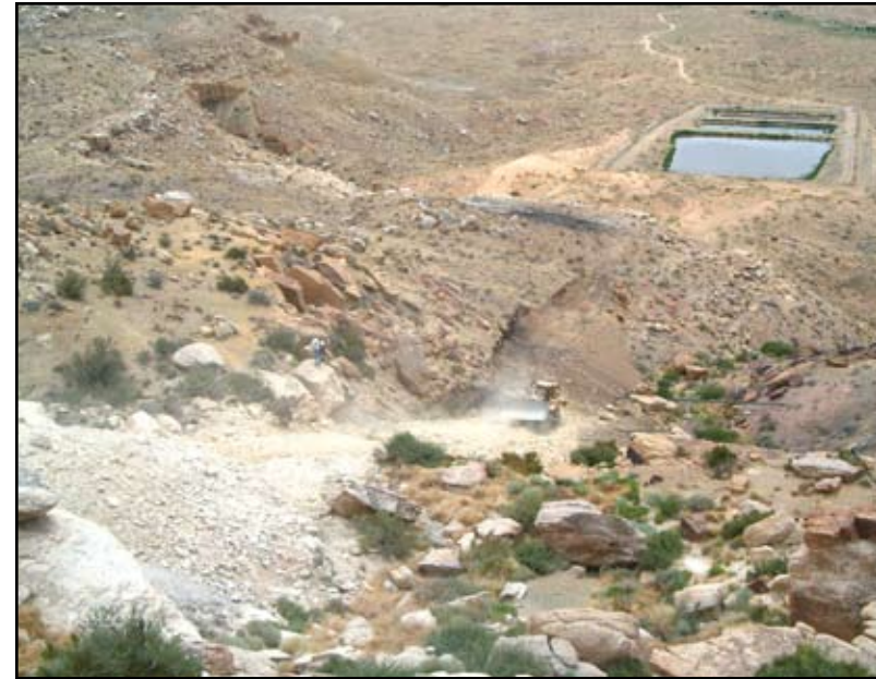
Figure 32: Completed wastewater lagoon upgrade, Village of Shungopavi.
