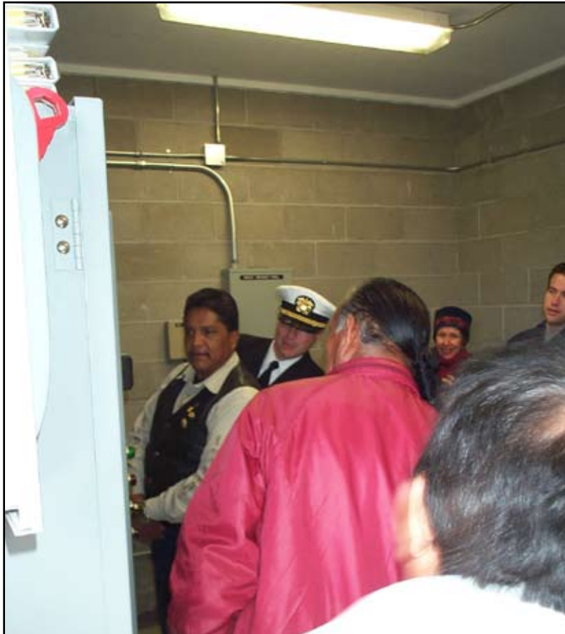
Figure 7: Governor of Santo Domingo Tribe turning on the well pump to send water to the Santo Domingo community for the “first” time.
