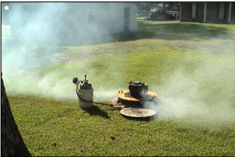
Figure 24: Smoke testing sewer mains at Chitimacha Reservation.
