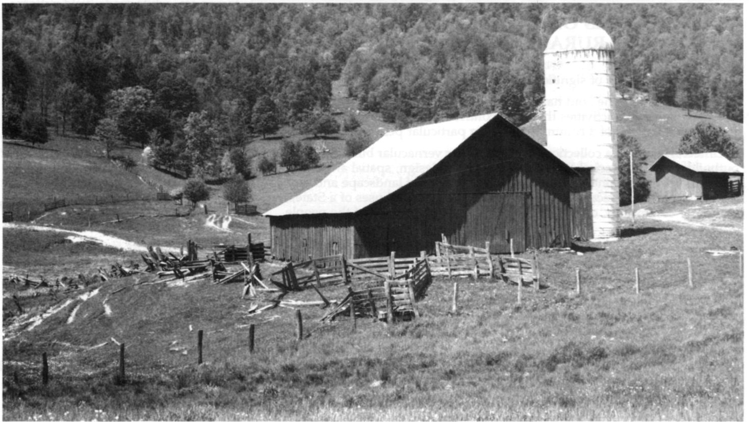
Setting is the physical environment within and surrounding a rural historic landscape. A fertile 40 square-mile basin atop 4,000-foot Garden Mountain, Burke's Garden Historic District, Tazewell County, Virginia, contains the material culture of occupations and agricultural activities from 8000 B.C. to the present. The district lies in the forested and sparsely settled highlands of the Southern Appalachians. (Virginia Department of Historic Resources)
