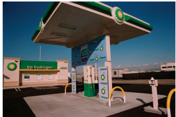
A hydrogen refueling station at Los Angeles International Airport.
