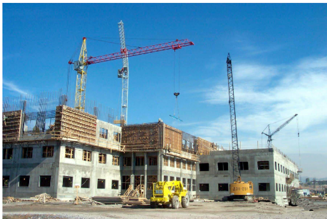
Ongoing embassy construction in Yerevan, Armenia.
