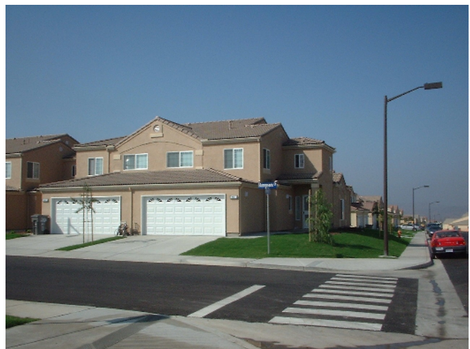
Family housing at Camp Pendleton, California.
