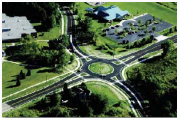
Figure 76. Aerial view of roundabout constructed in Michigan. (Photo courtesy of Wes Butch, DLZ Michigan, Inc.)
