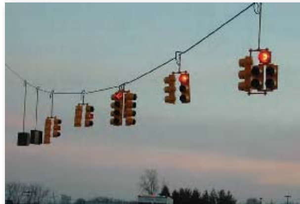
Figure 59d. Fourth set of signal indications when steady left red arrow is displayed.
