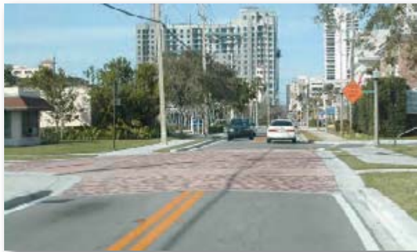
Figure 82. View of raised intersection/speed table in West Palm Beach.
