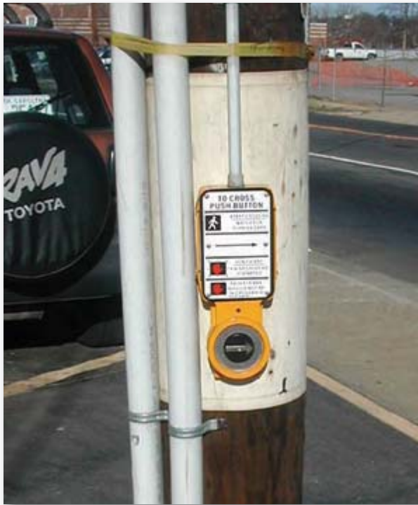
Figure 47. Pedestrian push button device in Charlotte with supplemental information in Braille on sign.
