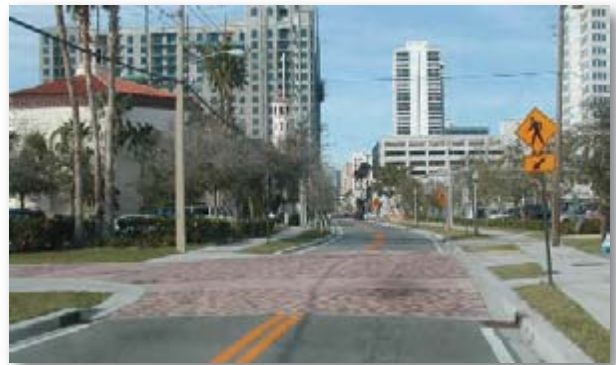
Figure 83. Closer view of raised intersection/speed table in West Palm Beach.
