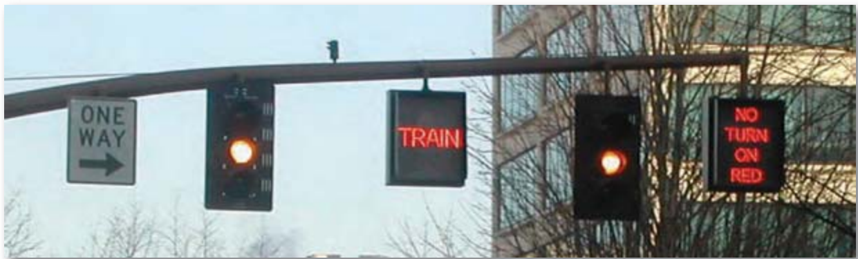
Figure 14. Dynamic regulatory and information signs used in Portland at an intersection where a trolley line crosses.
