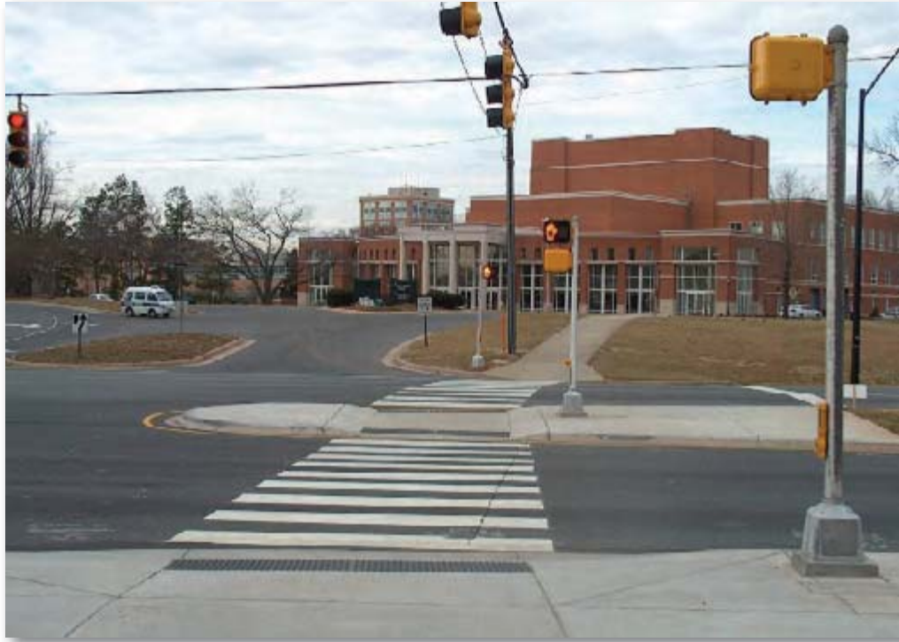
◀ Figure 95. Depiction of completed intersection geometric treatment implemented in Charlotte. (Courtesy of Charlotte DOT).
