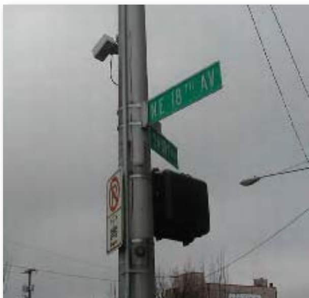
Figure 52. Pedestrian detection system that detects pedestrians in crosswalk in Portland.
