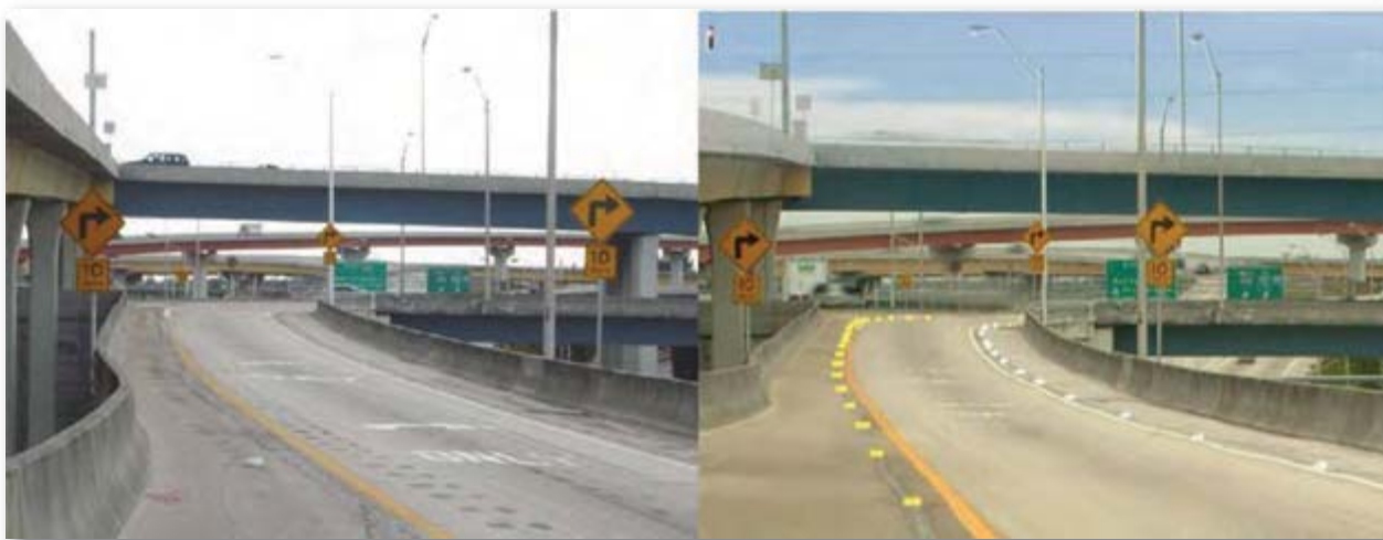
Figure 31. Two views of SR 84 off ramp before (left) and after (right) installation of LED modules. Note: Roadway conditions before and after LED modules installation. (Photo courtesy of Gilbert Soles, Florida DOT District 4).
