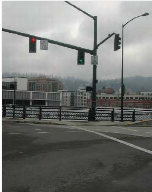
Figure 57. Signal heads and phasing for bicycle movement at intersection where video cameras are used in Portland.
