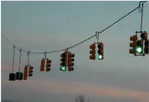
Figure 59c. Third set of signal indications when steady left green arrow is displayed.
