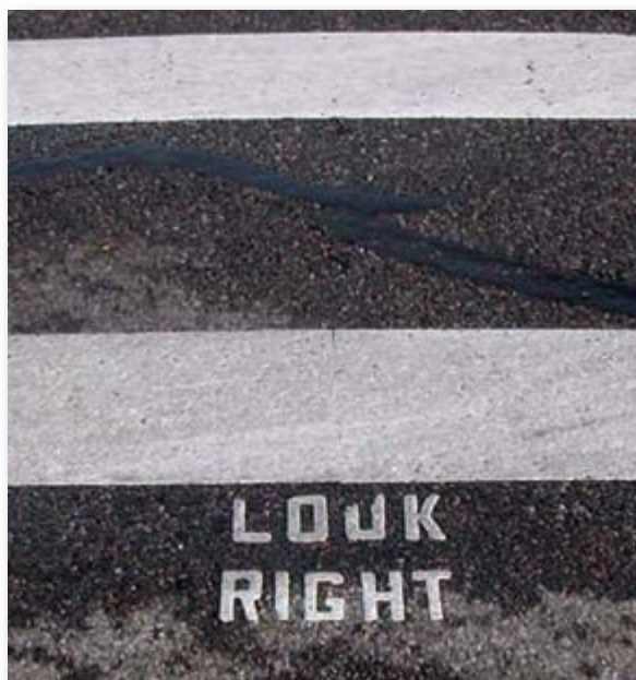
Figure 24. Pavement message for pedestrians at crosswalk.
