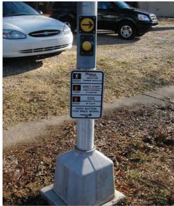
Figure 48. Example of another pedestrian push button device with supplemental raised arrow device mounted above the push button.
