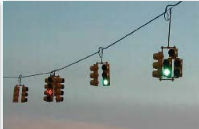
Figure 59b. Second set of signal indications when flashing yellow left arrow is displayed.
