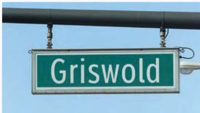
Figure 18. Overhead, internally illuminated street name sign with 12" letters in Clearview font (Photo courtesy of Kimberly Lariviere, Michigan DOT).
