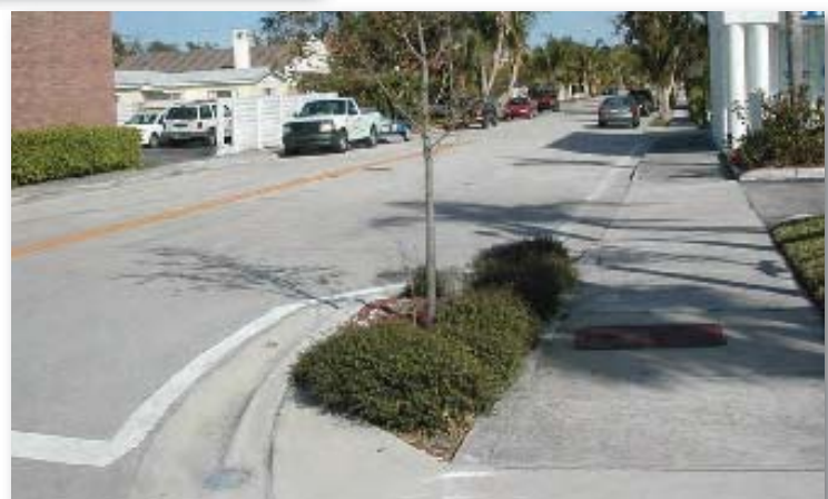
Figure 68. Intersection bulb-outs to define parking lane in a commercial area of West Palm Beach. ▶
