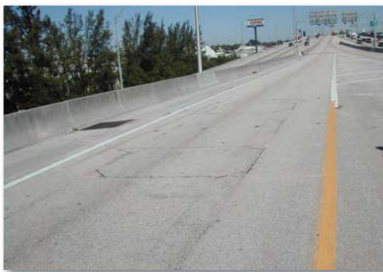
Figure 30. Loops used for speed detection near "beginning" ramp upstream of sharp curve.
