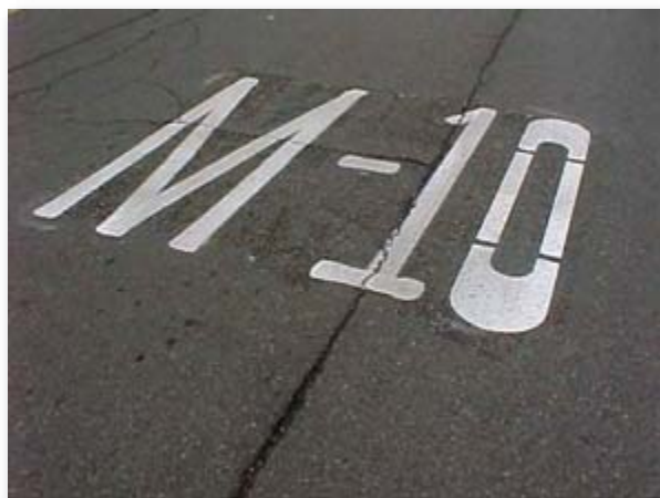
Figure 23. In-lane pavement marking message designating Michigan State Route 10 (M-10) applied in advance of an exist ramp.
