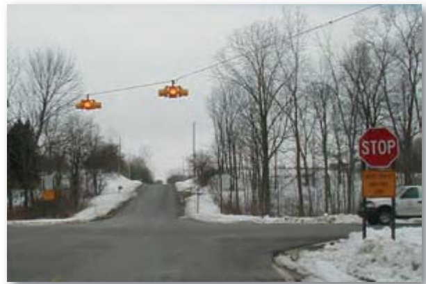
Figure 21. Signing treatment for two-way stop controlled intersection. (Photo provided by Tim Haagsma, Kent County Roads Commission).
