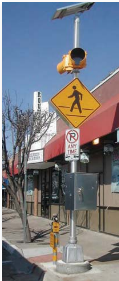
Figure 42. Activated flashing beacon that complements static warning sign and in-pavement crosswalk lights in Dallas.
