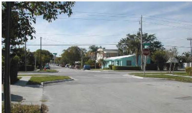
◀ Figure 67. Intersection bulb-outs to reduce the street width opening in a residential area in West Palm Beach.
