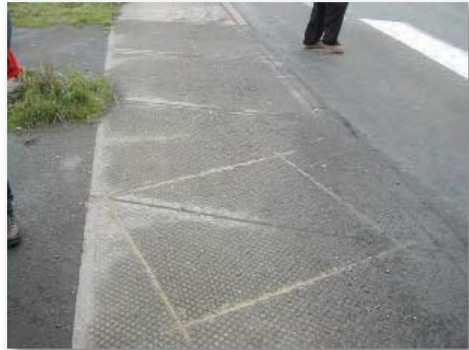
Figure 54. Loop in trail crossing to detect bicyclists in Portland.
