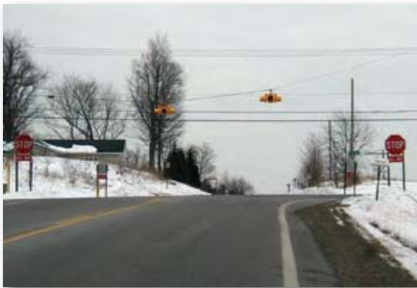
Figure 20. Signing treatment for all-way stop controlled intersection. (Photo provided by Tim Haagsma, Kent County Roads Commission).
