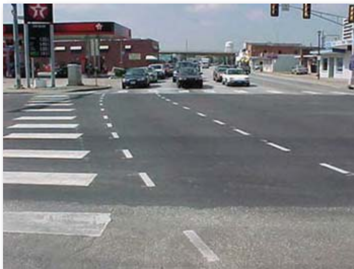
Figure 22. Intersection in Richardson with “cat” tracks, which are also called “puppy” tracks.
