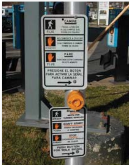
Figure 49. Pedestrian push button signs in both English and Spanish at an intersection in Charlotte.
