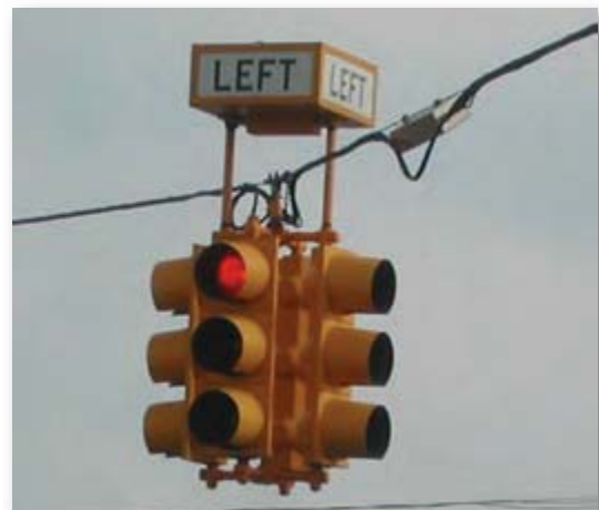
Figure 16. Overhead illuminated case “LEFT” sign in Michigan.
