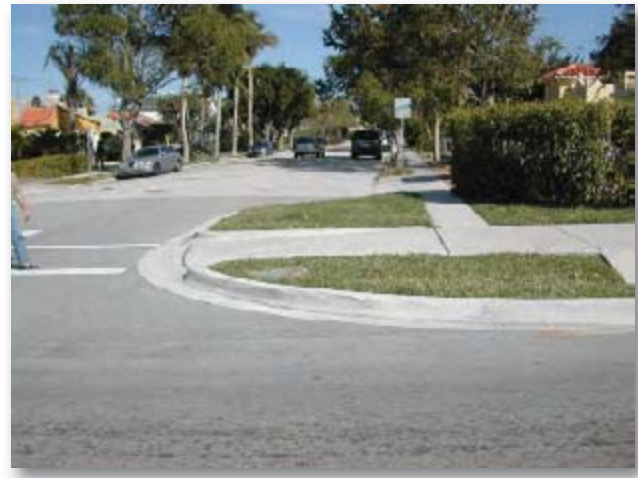
Figure 66. An example of an intersection “bulb-out” in West Palm Beach, Florida.
