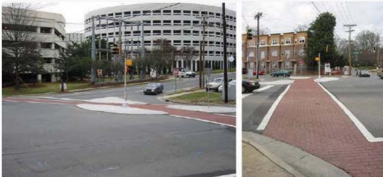
Figure 93. Two photographs of pedestrian refuge at an intersection in Charlotte after improvement. (Courtesy of Charlotte DOT).
