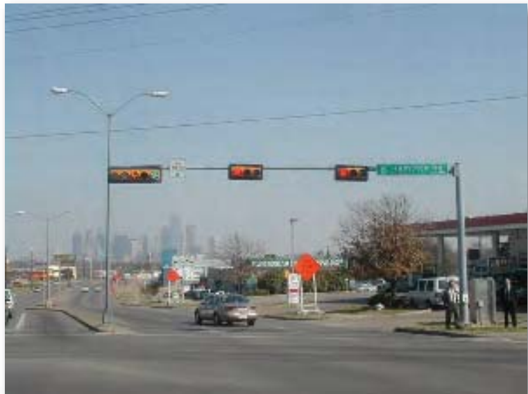
Figure 58. View from left-turn pocket where a Dallas (city in the background) phasing is in operation.
