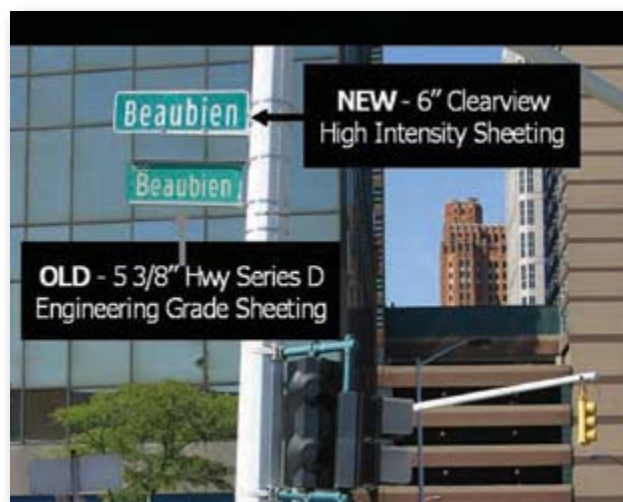
Figure 19. "OLD" and "NEW, improved" street name signs mounted on signal poles. (Photo courtesy of Kimberly Lariviere, Michigan DOT).
