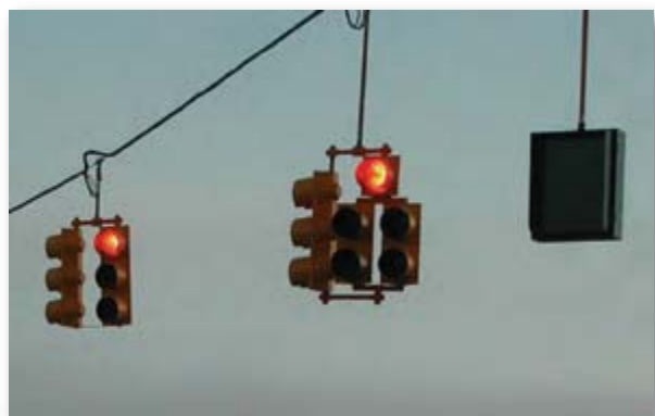
Figure 13. Dynamic regulatory sign at intersection in Michigan, with no message displayed (when a red left arrow is displayed to the opposing left turning traffic).
