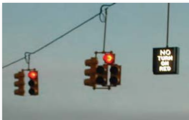
Figure 12. Dynamic regulatory sign at intersection in Michigan, with the “NO TURN ON RED” message displayed (when a left green arrow signal indication is displayed to opposing left turning traffic).
