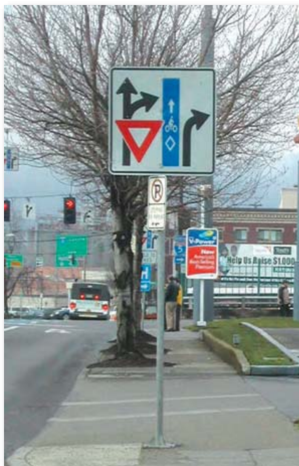
Figure 40. A regulatory sign for the situation where a blue bike lane “straddles” a dedicated right turn only lane and a shared-use, right-and-through lane.
