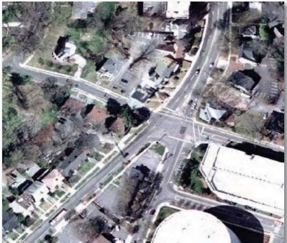
Figure 91. Aerial view of intersection in Charlotte prior to implementation of geometric treatment. (Courtesy of Charlotte DOT).
