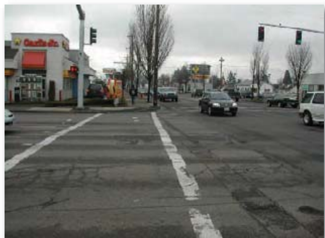
Figure 61. Intersection approach in Portland where loops beyond the stop line are used to delay the onset of the yellow interval.
