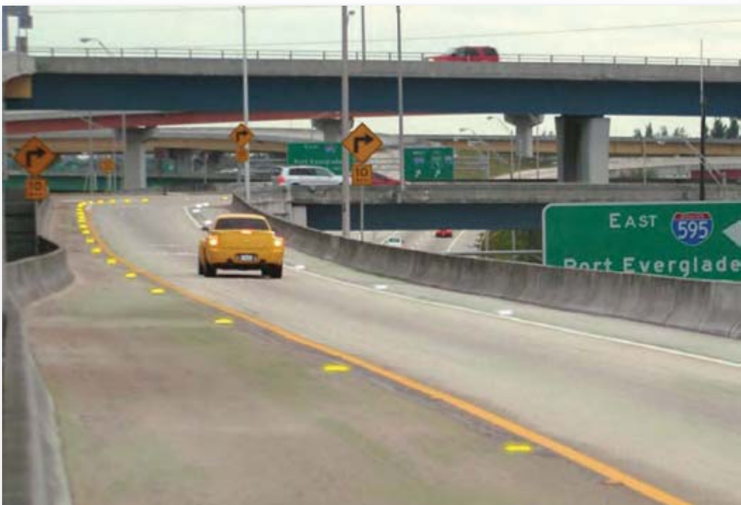
Figure 33. View of the system during daylight hours with the in-pavement lights “on.” (Photo courtesy of Gilbert Soles, Florida DOT District 4).
