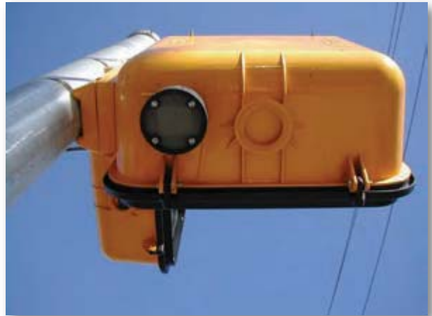
Figure 45. Speaker on underside of a pedestrian head in Charlotte.
