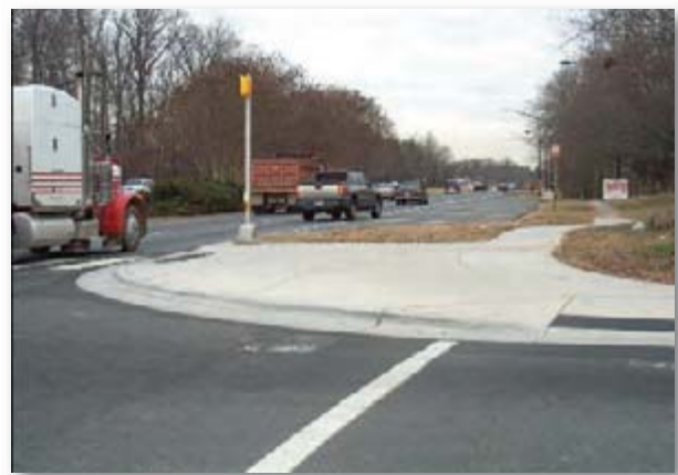
Figure 97. Close up of larger concrete landing in one corner. (Courtesy of Charlotte DOT).
