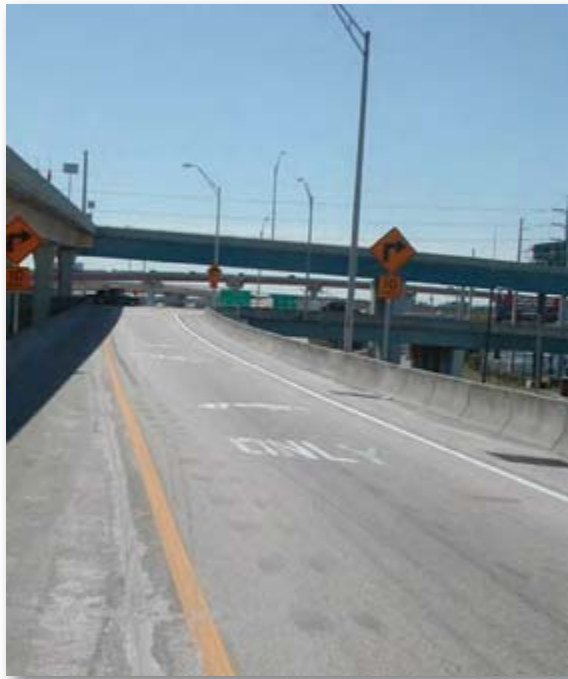
Figure 26. View of the ramp of in-pavement lighting device.
