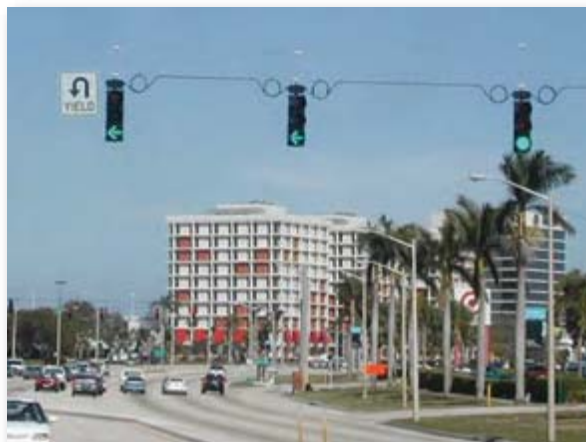
Figure 11. “U-TURN YIELD” regulatory sign for Left turn signal head on an approach with dual Left turn lanes in south Florida.
