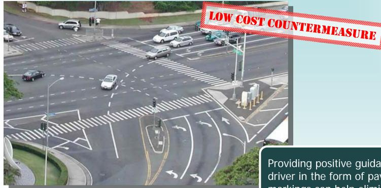
Providing positive guidance for the driver in the form of pavement markings can help eliminate driver confusion and eliminate vehicle conflict by channeling vehicles in their proper turn path.
