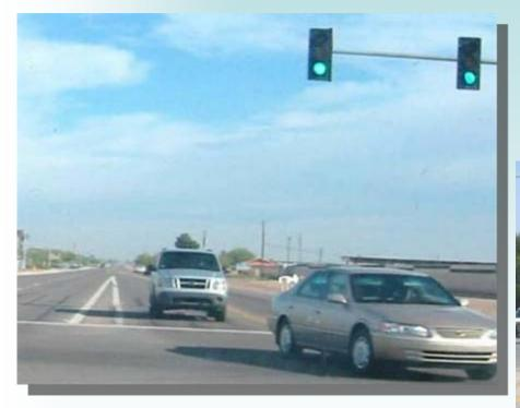
[Offset left turn lanes help] improve safety and operations of the left-turn movement by improving driver acceptance of gaps...
