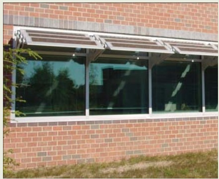
Photovoltaic window shades produce energy
