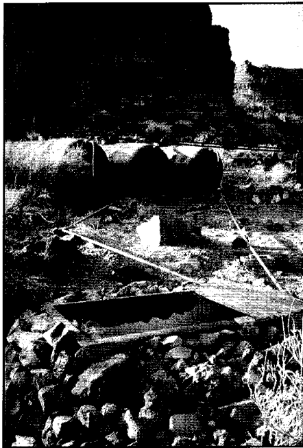
Red Cliff (Hwy 95) wildlife water catchment.
