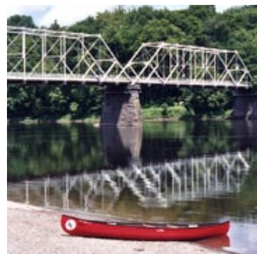
Dingmans Ferry Bridge 2004.
