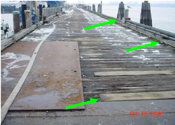
Highlight 12 shows the deck of Mallory Pier, the main training ship berthing pier. Metal plate covers large hole caused by rotten planks. Green arrows highlight (top to bottom) rusting 440v power terminal conduit; rotting power cable foundation; new planks installed to replace rotten planks over smaller holes.
