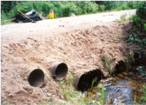
A typical eroding culvert crossing in the Salmon Trout River Watershed Photograph by Joe Wagner
