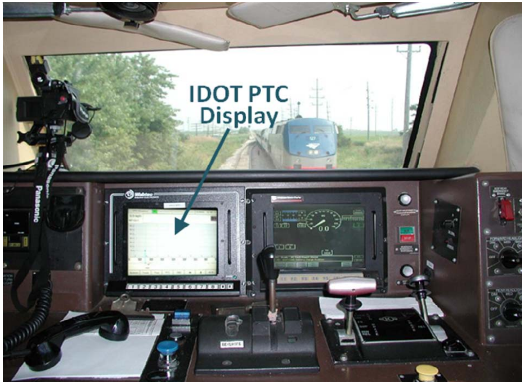
Figure A-1. NAJPTC Display Installed in a P42 Passenger Locomotive
