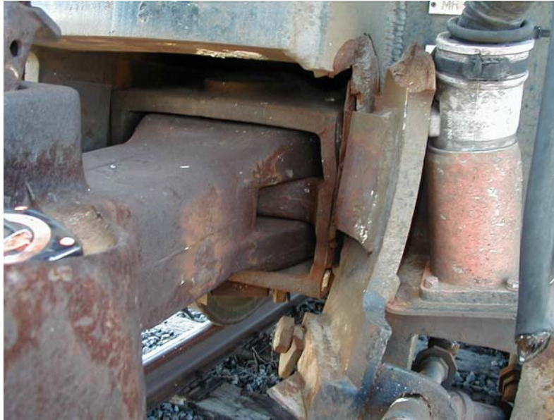
Figure 10. Damaged Coupler Pocket of the Locomotive
