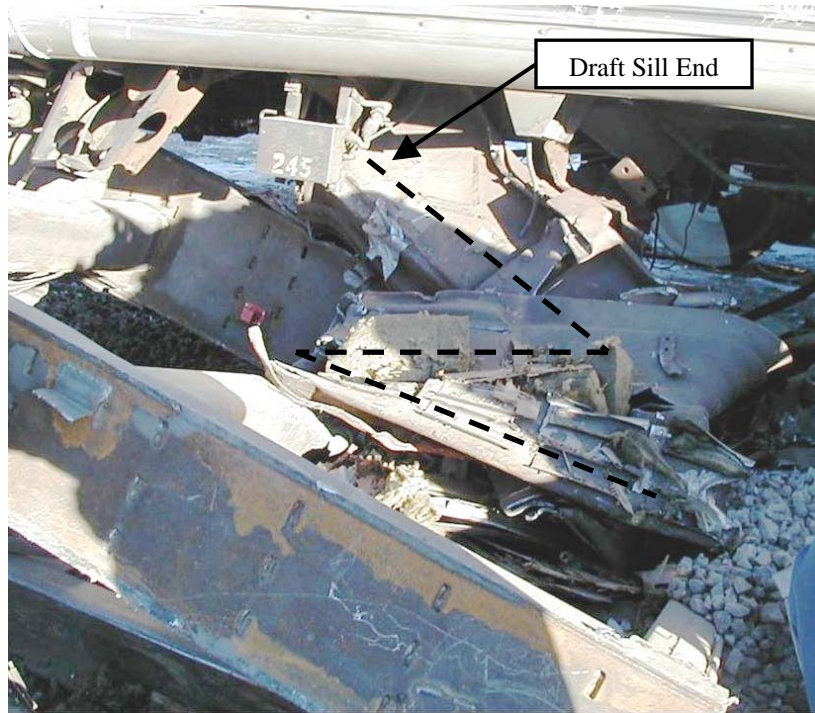
Figure 13. Photograph of Deformed Draft Sill (Dashed Line Shows Bent Shape of the Draft Sill)
