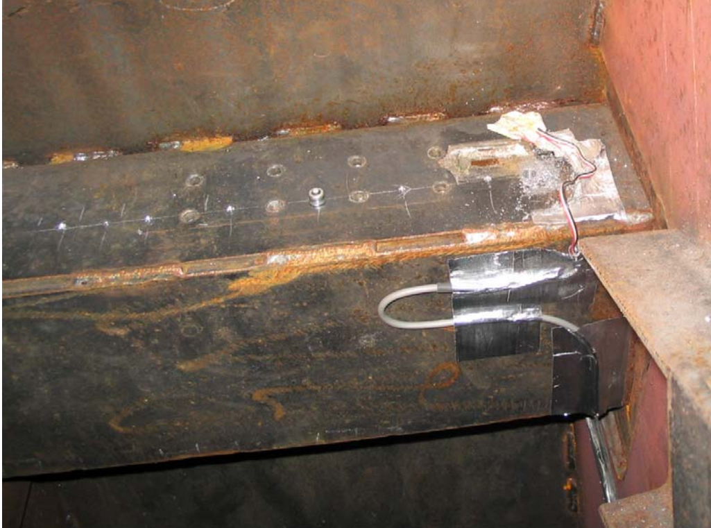
Figure 27. Rivet Pattern for the Repaired Roof Absorber Shear Joint (Top Surface)
