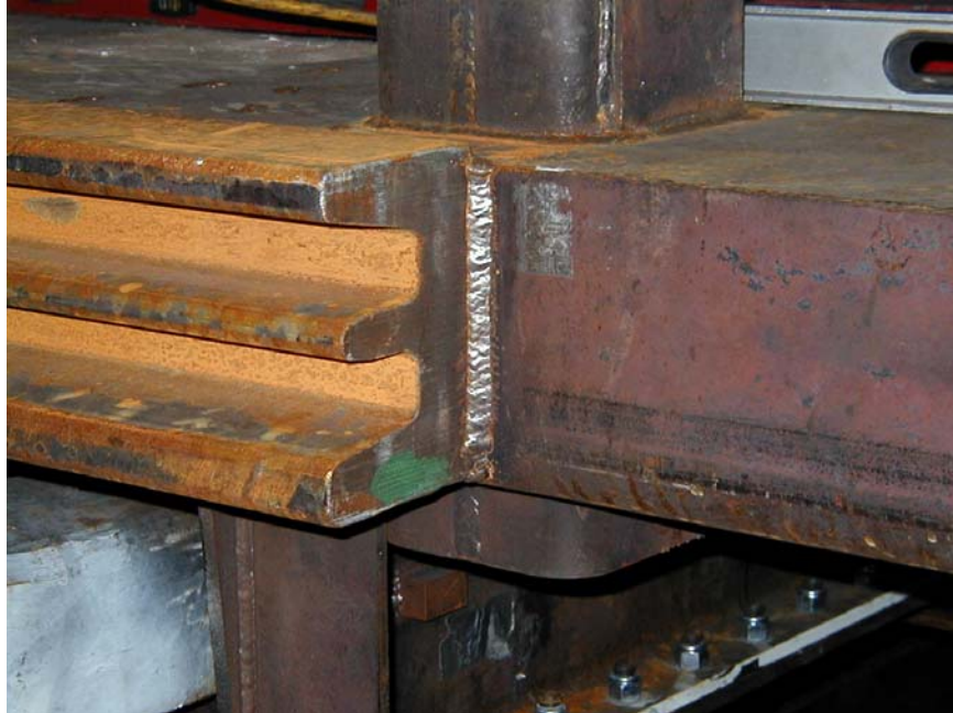
Figure 17. Anticlimber with Chamfered Edge Welded to the End Beam
