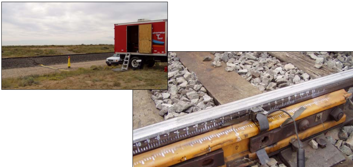
Figure 33. (Top) PA System Setup at FAST; (Bottom) Field Side Location of PA Transducer on Railhead
