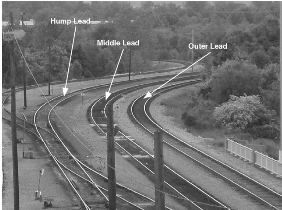
Figure 13. RCL1 southward view of outer, middle, and hump lead tracks and regular crossover in the foreground
