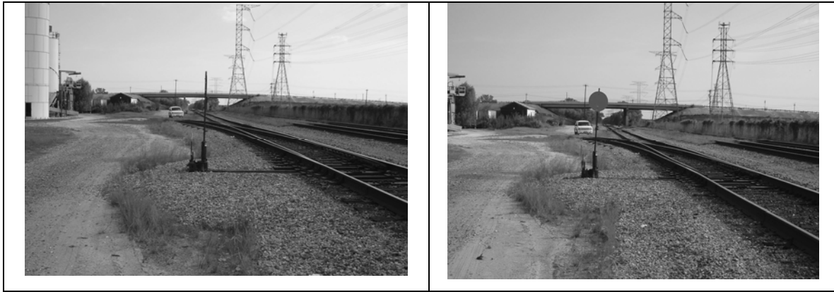
Figure 54. RCL5 industrial lead switch target communicating straight (trim 2) track movement (left) and industrial lead movement (right)
