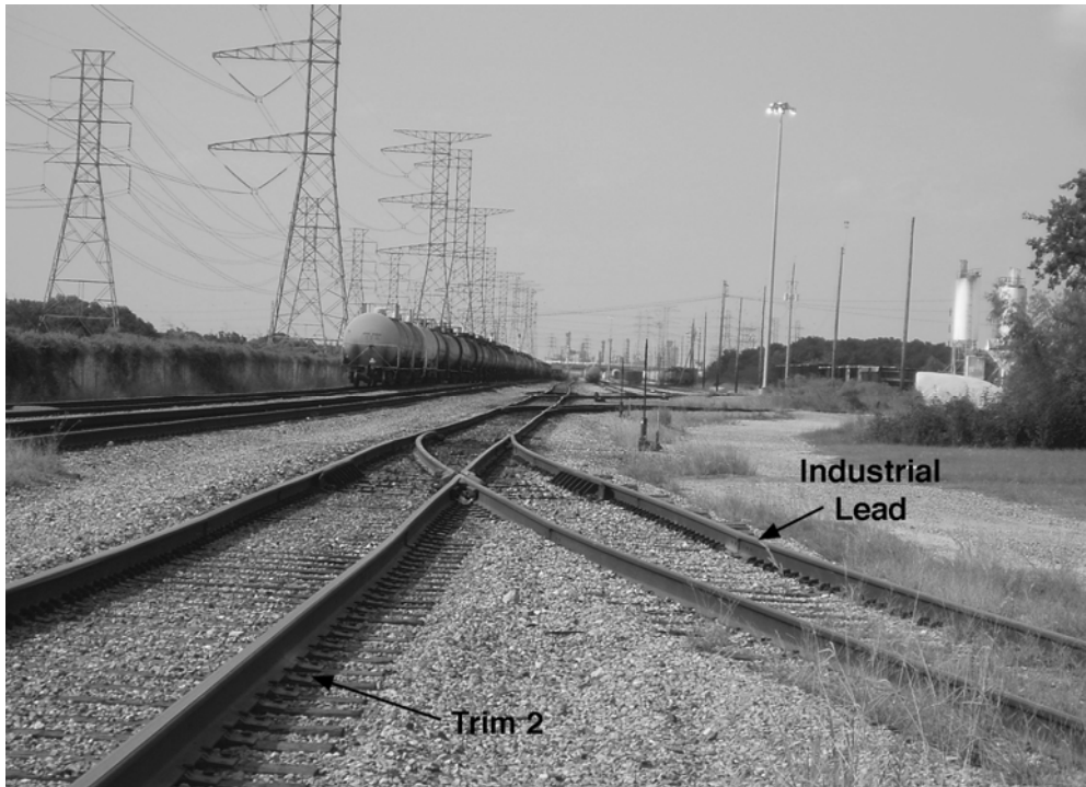
Figure 51. RCL5 northward view of trim 2 and industrial lead tracks
