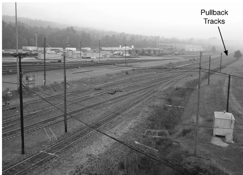
Figure 62. RCL6 view of crossovers at the south end of pullback tracks near yardmaster office
