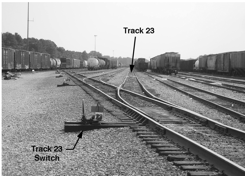
Figure 38. RCL4 view of ladder and track 23
