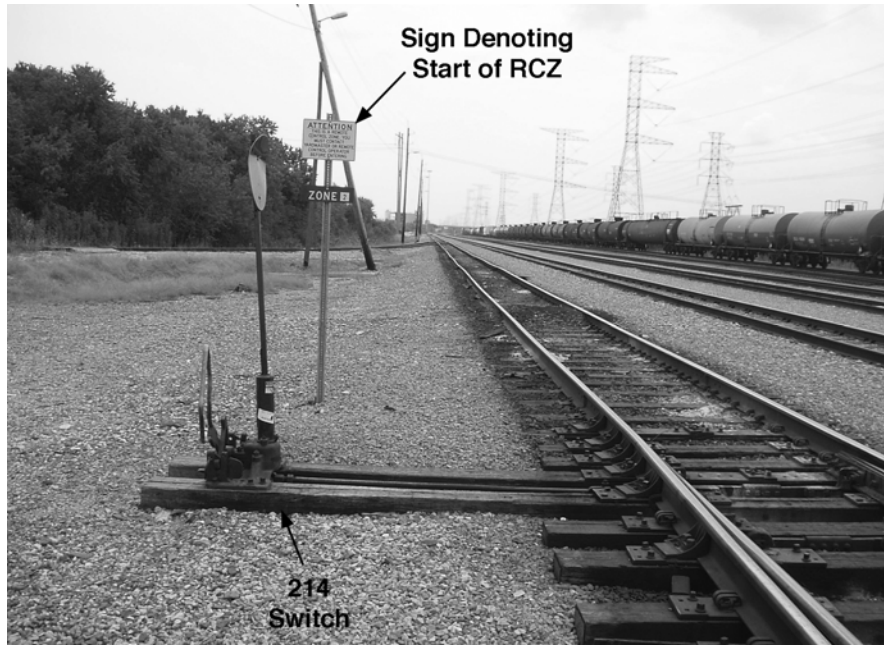
Figure 49. RCL5 southward view of 214 switch and start of RCZ along trim 2 track
