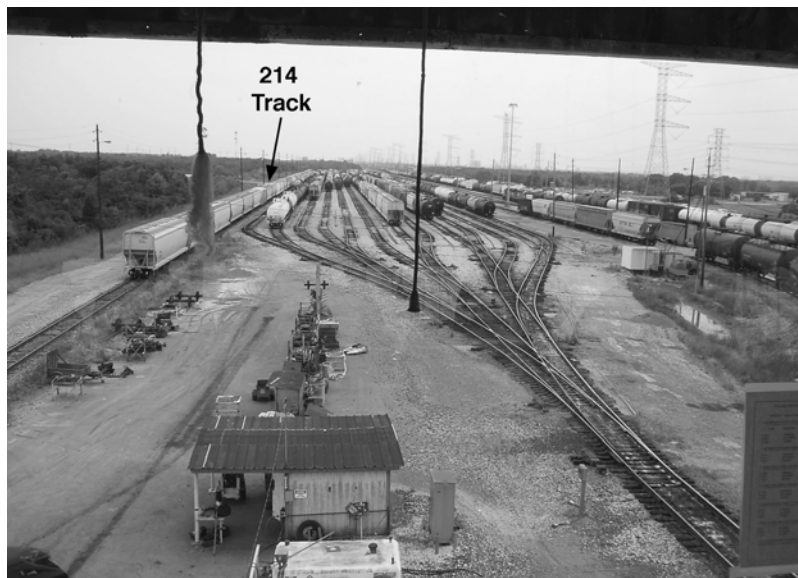
Figure 48. RCL5 southward view of bowl tracks and 214 track from hump tower
