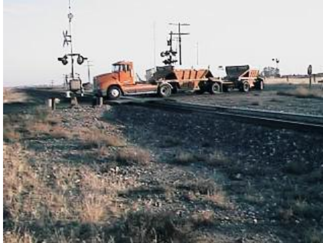
Figure 4. Rural Crossing Along the Study Area
