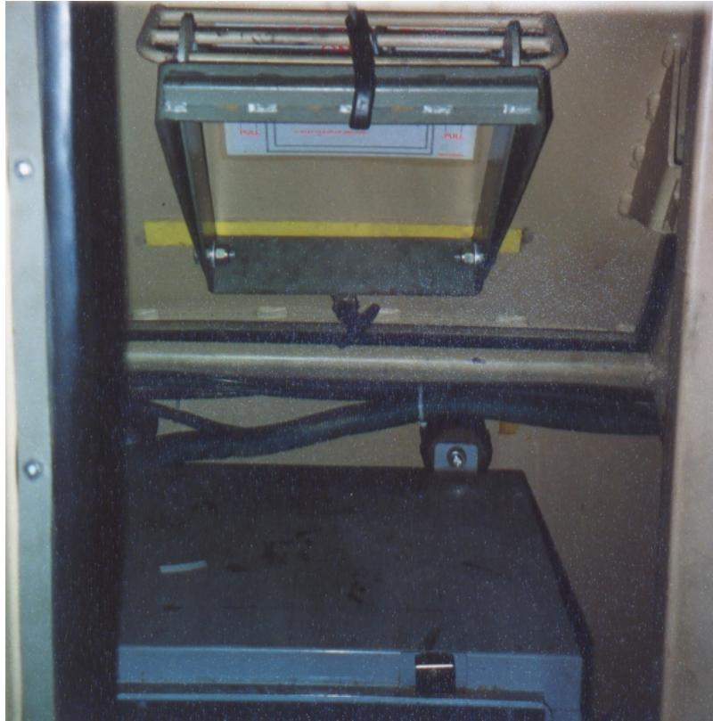
Figure 11. Interior view of nose hatch (refrigeration unit located below)
